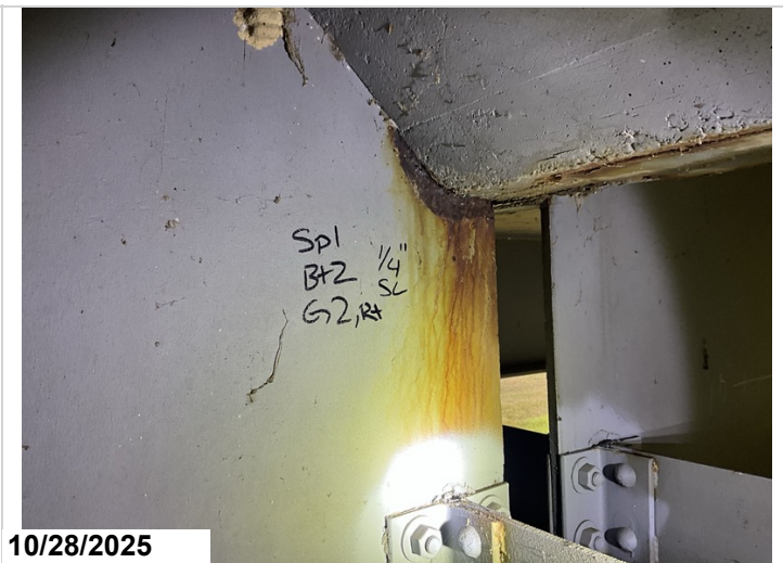
Span 1, Bent 2, Girder 2, Right: Active corrosion with section loss up to 1/4" to the web at the haunch area. 1LF CS3 corrosion.
