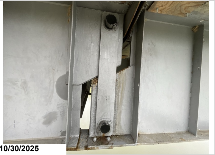
Span 8, First set of Pin and Hanger Assembly's: Pin and Hanger Assembly's have been replaced since the last inspection.
