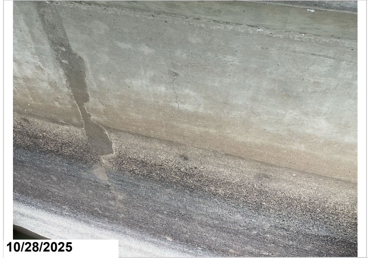
Pier 3, Back, Wall: Vertical cracking Right of centerline. 1LF CS2 cracking.
