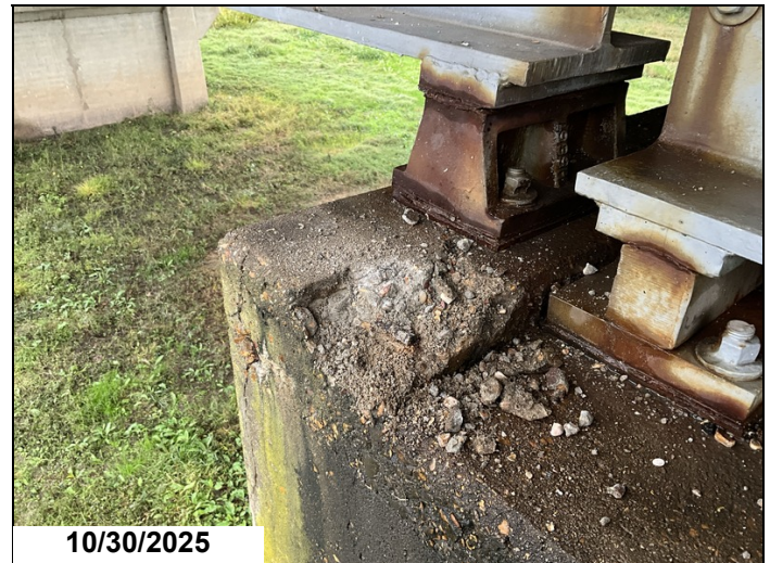
Bent 6, Left: Spalling with exposed reinforcing steel with section loss. 1LF CS3 exposed reinforcing steel.
