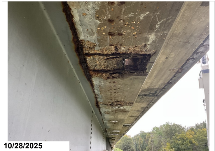
Span 6, Right overhang: Spalling with exposed reinforcing steel with section loss. 7SF CS3 exposed reinforcing steel.
