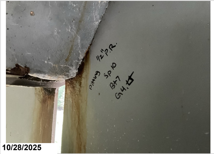
Span 10, Bent 7, Girder 4, Left: Active corrosion with pack rust up to 1/2" between the girder web and the concrete haunch. 1LF CS3 corrosion.
