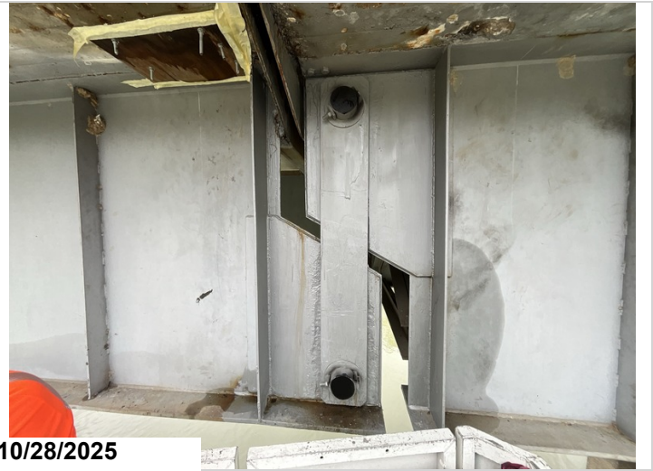
Span 8, Second Pin and Hanger Assembly's: Pin and Hanger Assembly's have been replaced since the last inspection.
