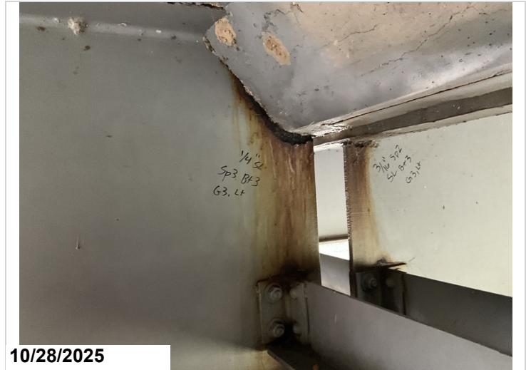
Span 3, Bent 3, Girder 3, Left: Active corrosion with section loss up to 1/4" to the web at the haunch area. 1LF CS3 corrosion.
