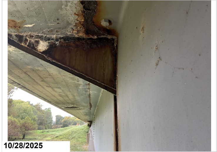
Span 6, Bent 6, Girder 4: Distortion in the web due to pack rust between the Girder web and the concrete haunch.
