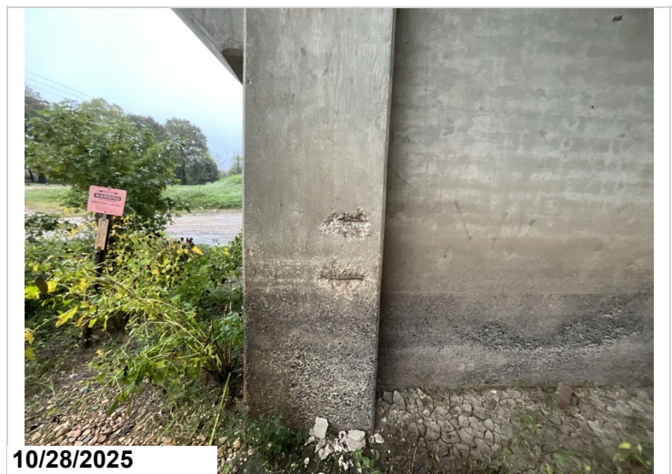
Pier 4, Column 1, Back: Spalling with exposed reinforcing steel. 1EA CS3 exposed reinforcing steel.
