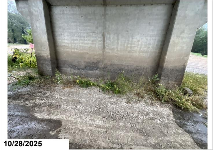
Pier 4, Wall, Ahead and Back: Abrasion from ground line to 3' above ground line. Rest in CS2 Abrasion.
