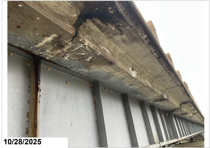
Span 8, Left overhang: Cracking with efflorescence. 14sf CS3 efflorescence.
