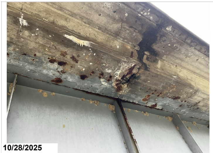
Span 8, Left overhang: Spalling with exposed reinforcing steel with section loss. 12SF CS3 exposed reinforcing steel.
