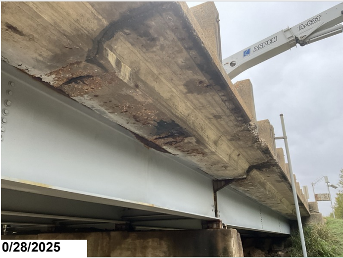
Span 10, Right overhang: Spalling with exposed reinforcing steel with section loss. 8SF CS3 exposed reinforcing steel.
