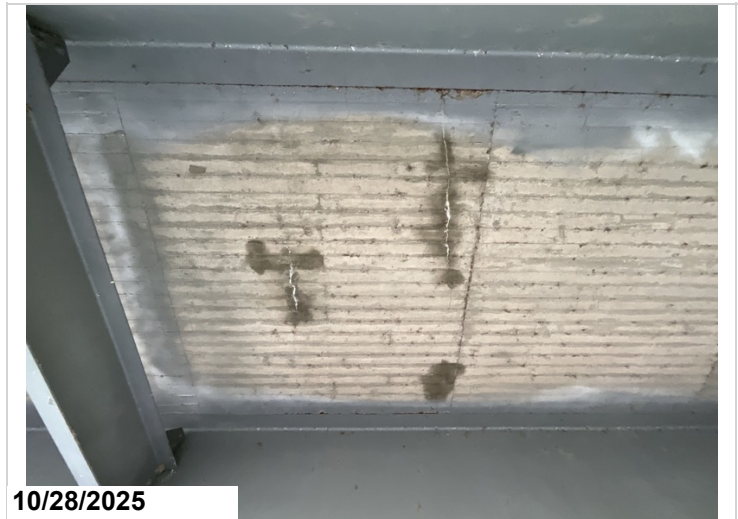
Span 4, undersurface: Cracking with efflorescence. 32sf CS2 efflorescence.
