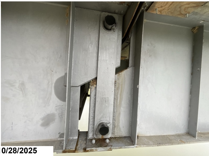
Span 8, First set of Pin and Hanger Assembly's: Pin and Hanger Assembly's have been replaced since the last inspection.
