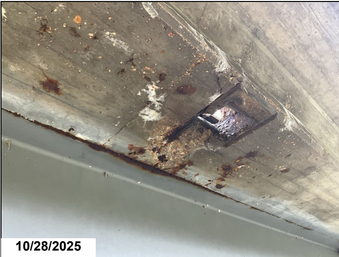
Span 4, Right overhang: Spalling with exposed reinforcing steel at the drains. 2SF CS3 exposed reinforcing steel.
