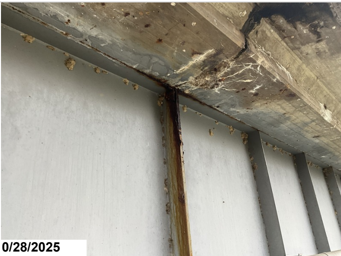
Span 9, Pier 3, Girder 1, Left: Active corrosion with flaking rust along the Top Flange. 4LF CS3 corrosion.
