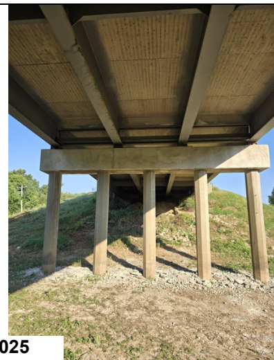
Bent 2 Cap: Repaired w/Galvanic Anodes
