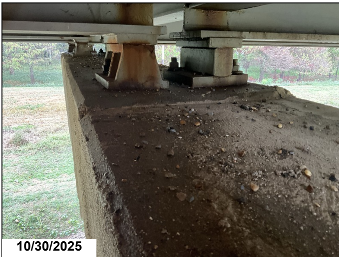
Bent 4, bearings.
