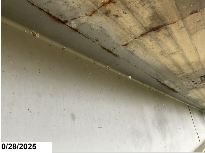
Span 5, Girder 1, Left: Active corrosion with flaking rust along the Top Flange. 10LF CS3 corrosion.
