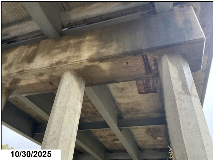
Bent 7, Cap: Spalling with exposed reinforcing steel with section loss. 8LF CS3 exposed reinforcing steel.
