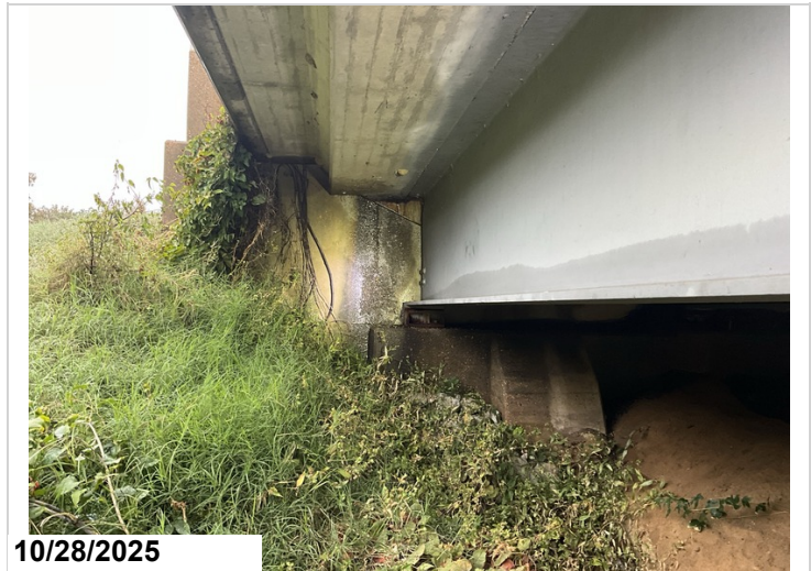
Bent 1, behind Girder 4, Backwall: Spalling. 1LF CS3 Spalling.
