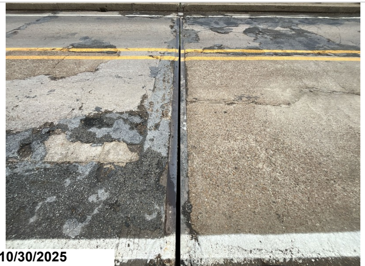
Bent 7, Joint: Armor missing for the full length. 26LF CS4 metal deterioration.
