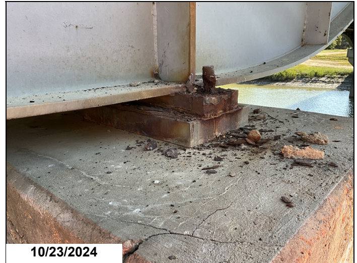
Corrosion with pack rust typ all bearings.
