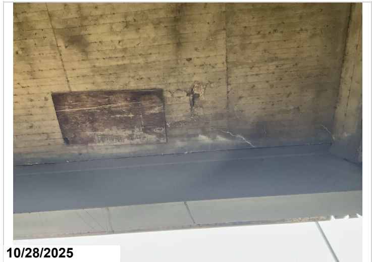
Span 11, Bay 3, Ahead of Bent 7: Spalling with exposed reinforcing steel with section loss. 1SF CS3 exposed reinforcing steel.
