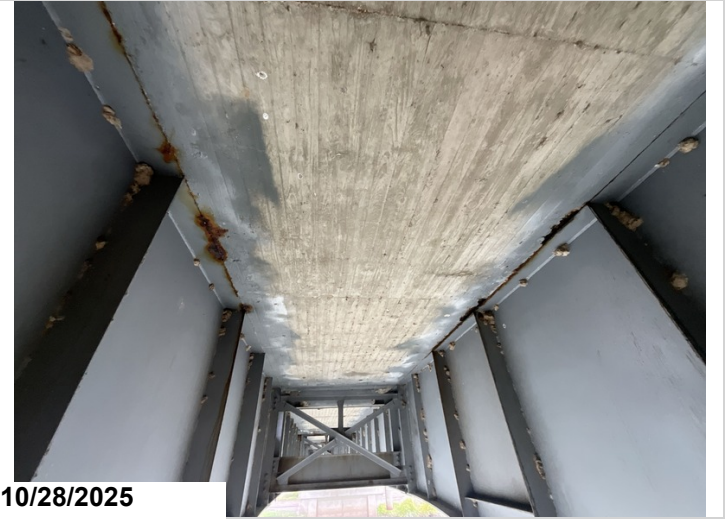
Span 8, Girders 1 and 2: Active corrosion with flaking rust along the Top Flange. 8LF CS3 corrosion.
