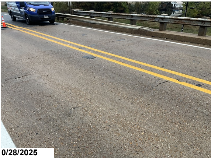
Span 1: Transverse cracking. 71SF CS3 cracking.
