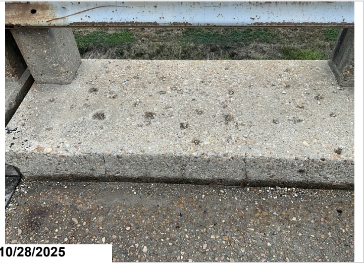
Multiple transverse cracks in curbs.
