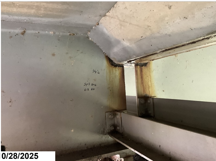
Span 5, Bent 6, Girder 2, Right: Active corrosion with section loss up to 1/4" to the web at the haunch area. 1LF CS3 corrosion.
