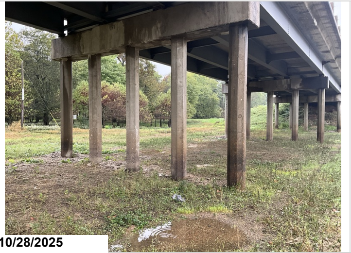
Bent 4, Piles 1 - 5: Minor abrasion. 5EA CS2 abrasion.
