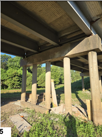
Bent 3 Cap: Repaired
