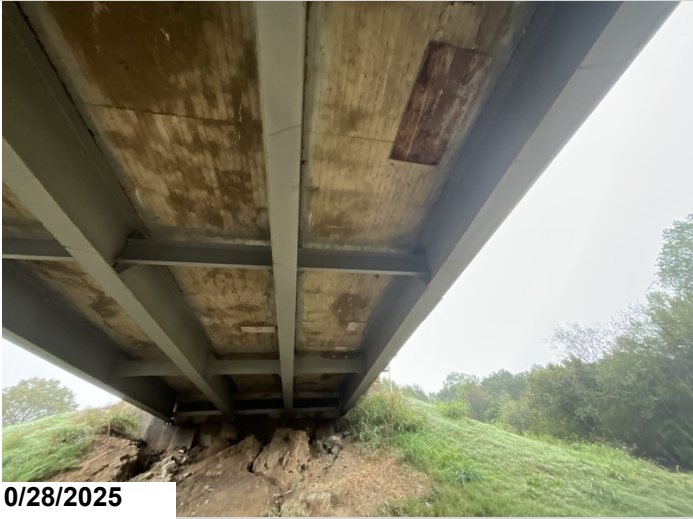
Span 11, Bays 2 and 3: Patched areas. 12SF CS3 Spalling.
