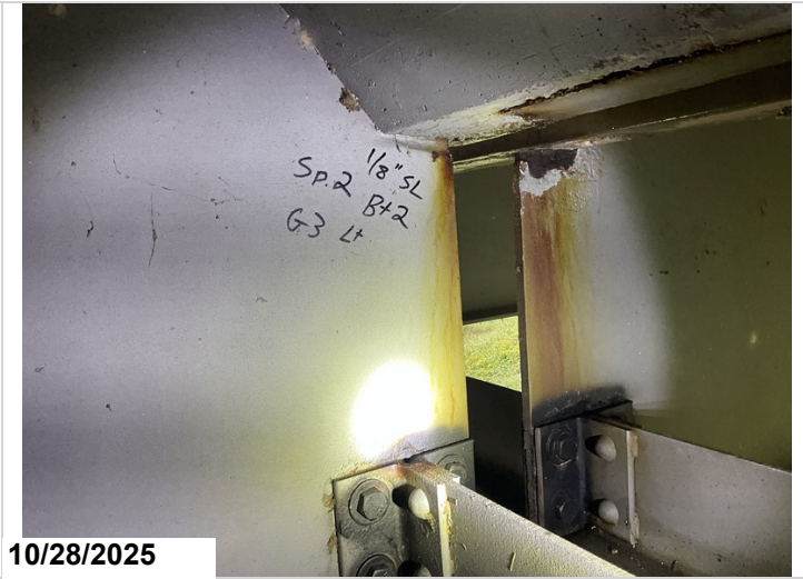
Span 2, Bent 2, Girder 3, Left: Old section loss scars up to 1/8". 1LF CS3 corrosion.
