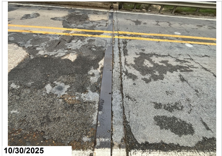
Bent 8, Joint: Debris impactation, full length. 26LF CS3 debris impactation.
