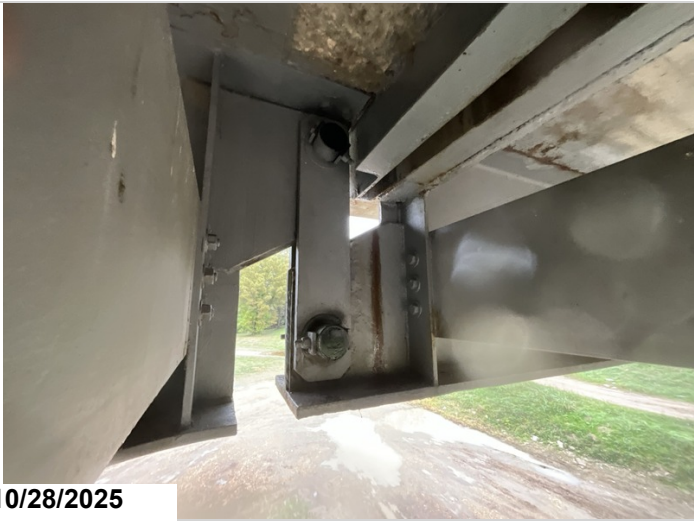
Span 10, Pin and Hanger Assembly: Pin and Hanger Assembly's have been replaced since the last inspection.
