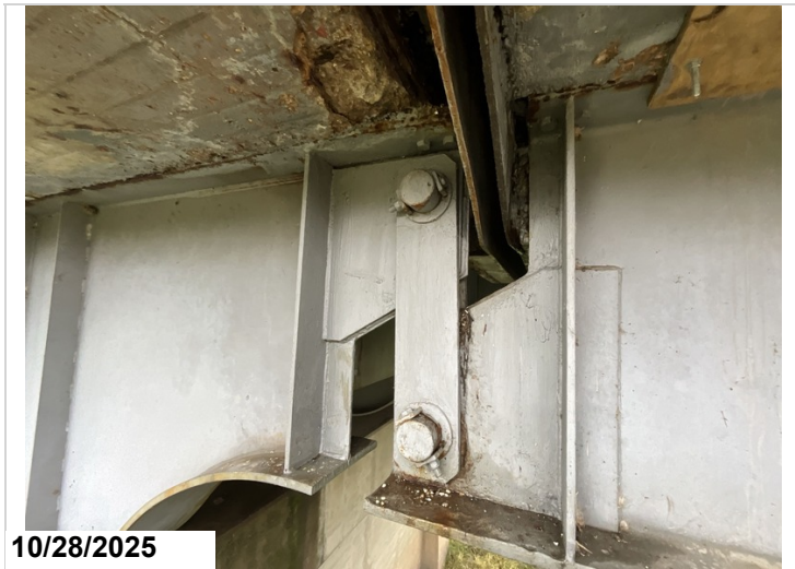
Typical Pin and Hanger Assembly.
