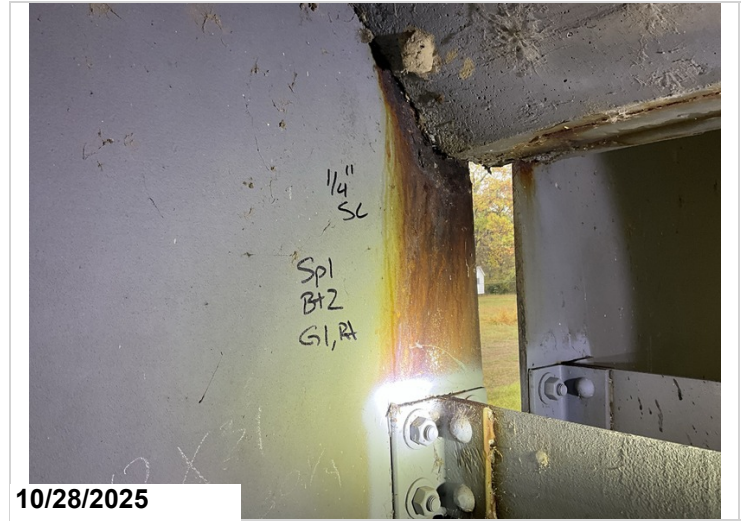
Span 1, Bent 2, Girder 1, Right: Active corrosion with section loss up to 1/4" to the web at the haunch area.
