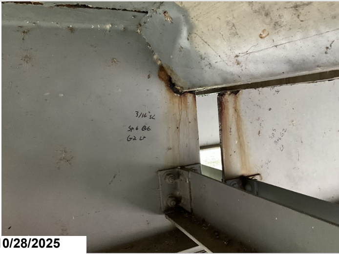
Span 6, Bent 6, Girder 2, Left: Active corrosion with section loss up to 3/16" to the web at the haunch area. 1LF CS3 corrosion.
