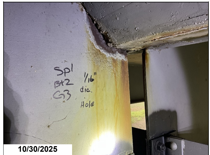
Span 1, Bent 2, Girder 3: Active corrosion with a 1/16" diameter hole in the web at the haunch area. 1LF cs4.
