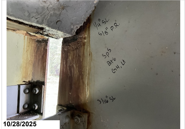
Span 5, Bent 6, Girder 4, Left: Active corrosion with section loss up to 1/4" to the web at the haunch area, section loss up to 3/16" to the web at the diaphragm connection, and pack rust up to 5/8" between the girder web and the concrete haunch. 1LF CS3 corrosion.
