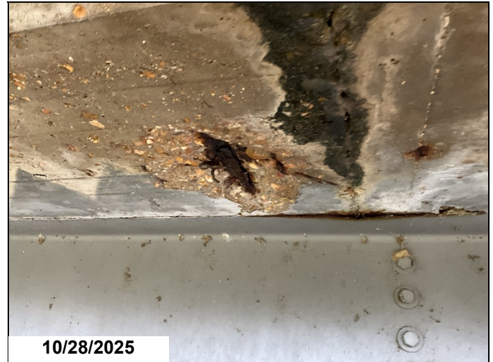
Span 10, Left overhang: Spalling with exposed reinforcing steel with section loss. 3SF CS3 exposed reinforcing steel.
