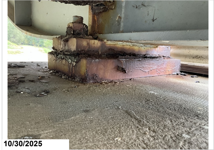
Pier 3, Bearings 1 - 4: Active corrosion with pack rust between the sole and masonry plate. 4EA CS3 corrosion.
