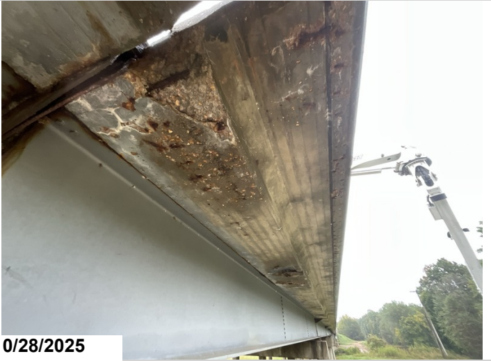
Span 3, Right overhang: Spalling with exposed reinforcing steel with section loss. 3SF CS3 exposed reinforcing steel.
