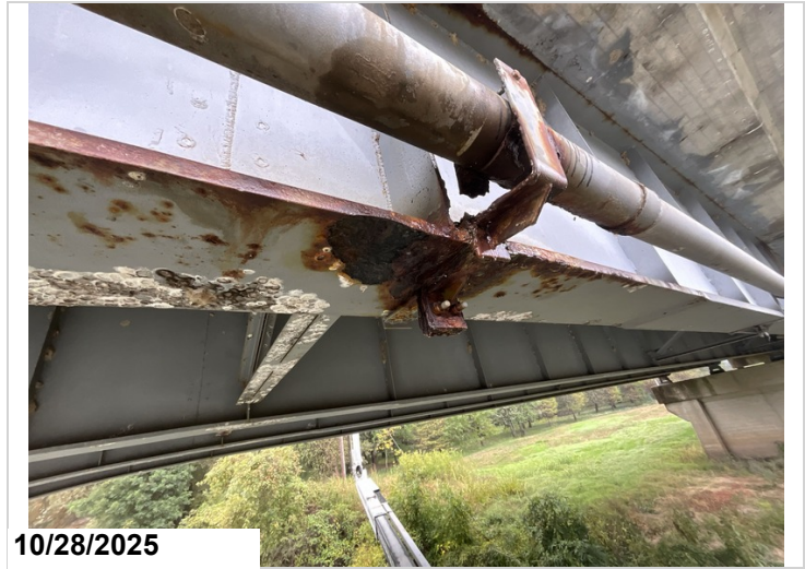
Span 7, Girder 1, Bottom Flange: Active corrosion with section loss up to 7/16" below the last saw joint before Pier 2.
