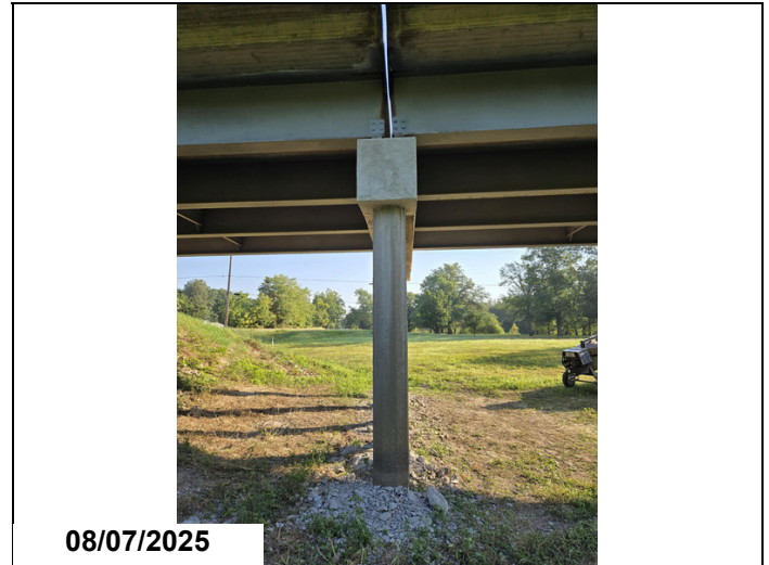
Bent 2 Cap: Repaired w/Galvanic Anodes
