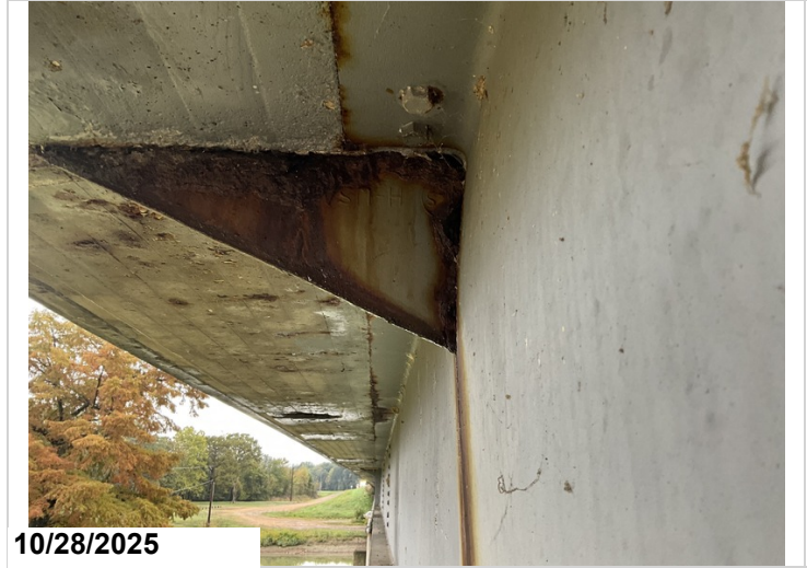
Span 5, Bent 6, Girder 1: Distortion in the web due to pack rust between Girder web and concrete haunch.
