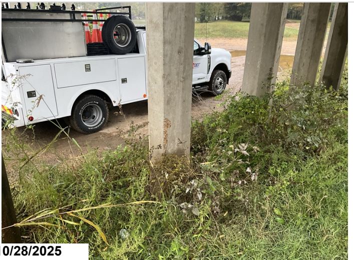
Bent 7, Pile 4: Minor spalling. 1EA CS2 spalling.
