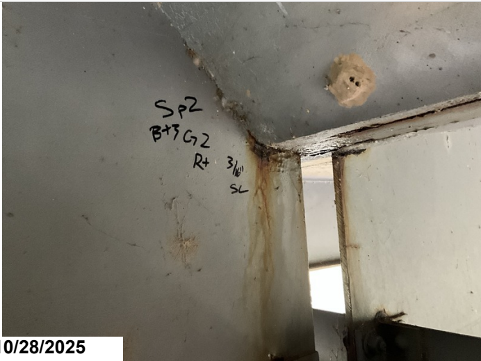
Span 2, Bent 3, Girder 2, Right: Active corrosion with section loss up to 3/16" to the web at the haunch area. 1LF CS3 corrosion.
