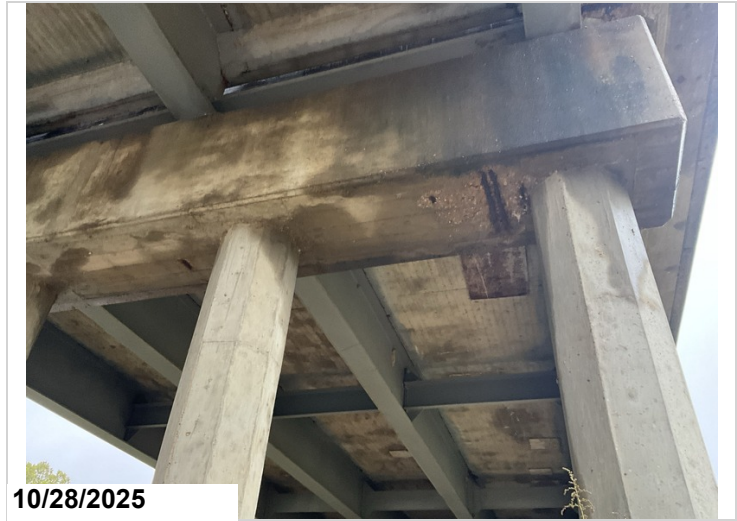
Bent 7, Cap: Spalling with exposed reinforcing steel with section loss. 8LF CS3 exposed reinforcing steel.
