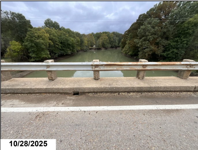
Span 8, Right: multiple post with cracking and spalling.
