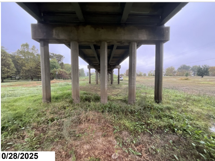
Bent 6, Piles 1 - 5: Minor abrasion. 5EA CS2 abrasion.
