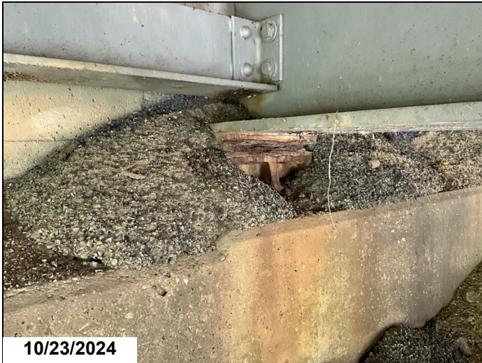
Bent 1, bearing 3: corrosion with severe pack rust raising girder elevation and severe asphalt debris accumulation around bearing. Typ at bearing 2. CS3 2 EA
