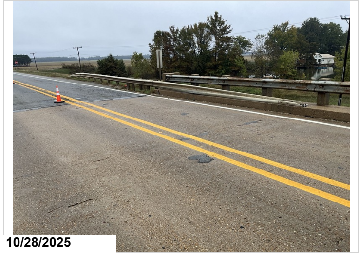
Span 1: Unsound patched and spalling. 28SF CS3 Spalling. Span 2: 26SF CS3 Spalling.
