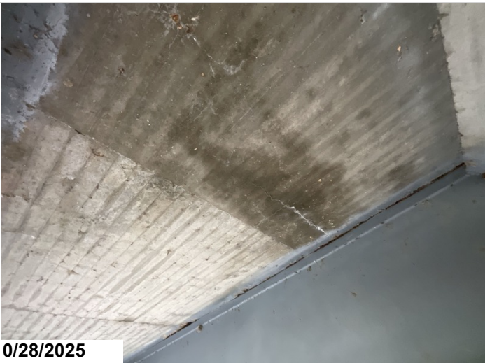
Span 3, All bays: 12SF CS2 efflorescence.
