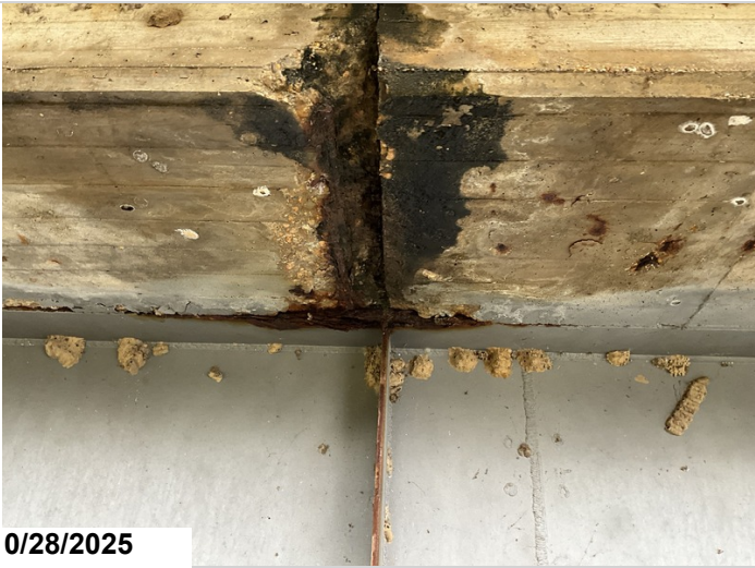
Span 9, Left overhang: Spalling with exposed reinforcing steel with section loss. 8SF CS3 Spalling.
