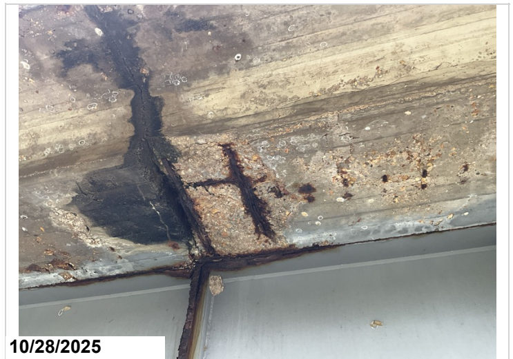
Span 8, Right Overhang: Spalling with exposed reinforcing steel with section loss. 10SF CS3 exposed reinforcing steel.
