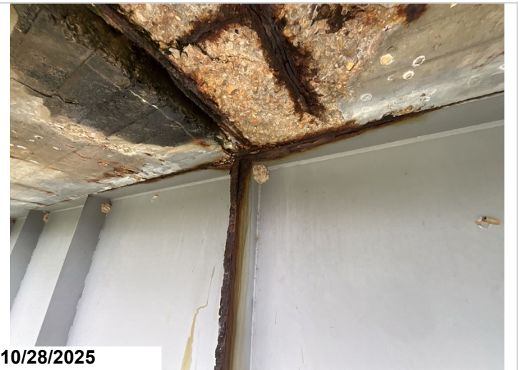
Span 8, Girder 4, Right: Active corrosion with flaking rust along the Top Flange and vertical bearing Stiffener. 6LF CS3 corrosion.
