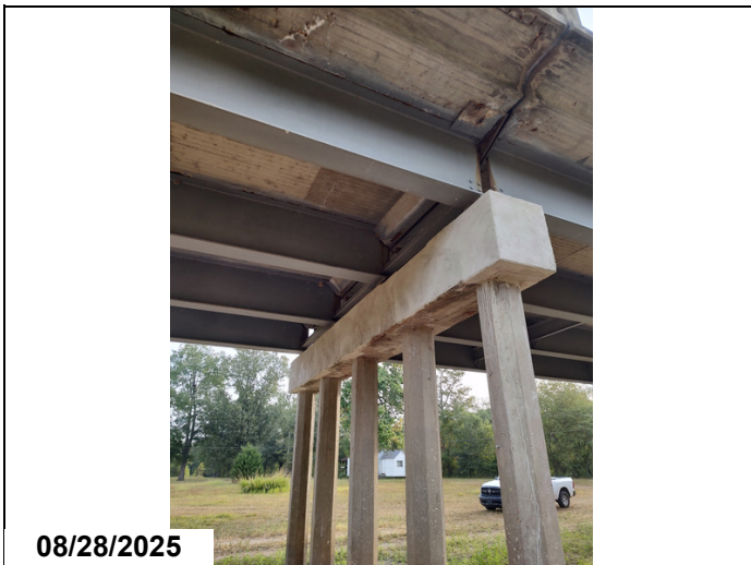
Bent 4, Cap: Repaired
