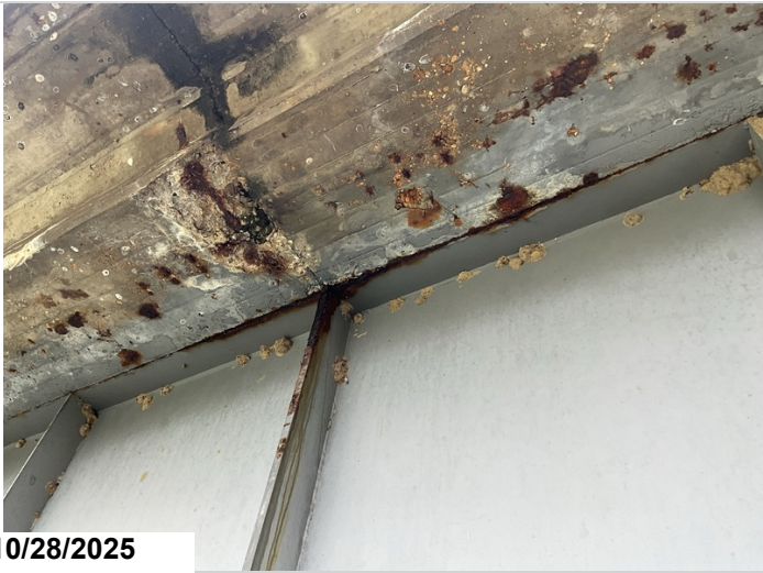
Span 7, Girder 1, Above Pier 2: Active corrosion with flaking rust along the Top Flange. 8LF CS3 corrosion.
