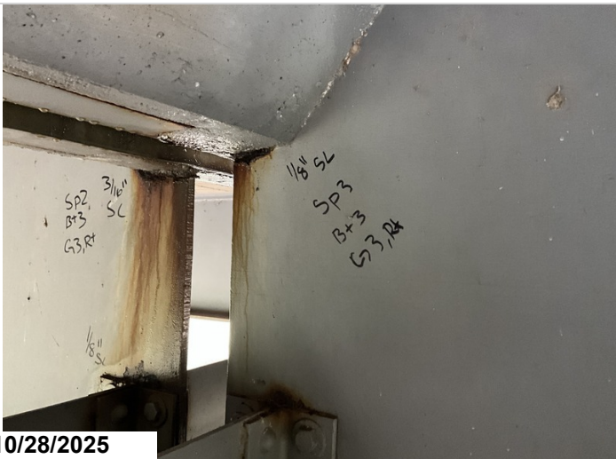
Span 3, Bent 3, Girder 3, Right: Active corrosion with section loss up to 1/8" to the web at the haunch area. 1LF CS3 corrosion.
