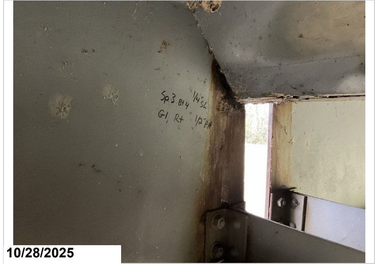
Span 3, Bent 4, Girder 1, Right: Active corrosion with section loss up to 1/4" to the web at the haunch area and pack rust up to 1/2" between the girder web and the concrete haunch. 1LF CS3 corrosion.
