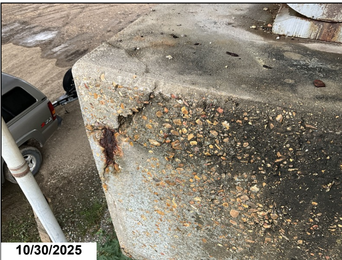
Pier 4, Left, Cap: Spalling with exposed reinforcing steel with section loss. 1LF CS3 exposed reinforcing steel.
