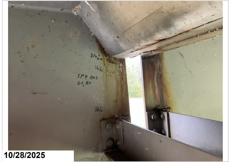
Span 4, Bent 5, Girder 1, Right: Active corrosion with section loss up to 1/4" to the web at the haunch area, section loss up to 1/8" to the web at the diaphragm connection, and pack rust up to 3/4" between the girder web and the concrete haunch. 1LF CS3 corrosion.
