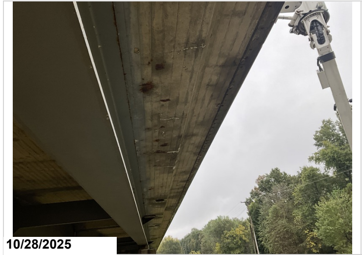
Span 3, Right overhang: 17SF CS3 efflorescence/rust staining.
