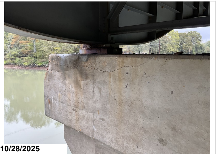
Pier 2, Cap, Back: Horizontal cracking between Girders 1 and 2. 7LF CS3 cracking. Ahead side mirrors.
