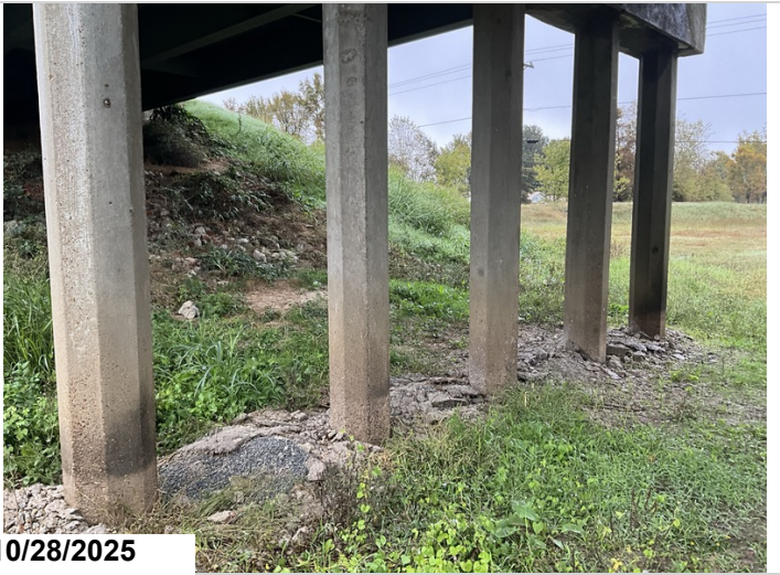
Bent 2, Piles 1 - 5: Minor abrasion. 5EA CS2 abrasion.
