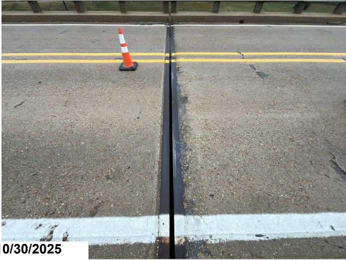
Bent 2, Joint: Armor missing for the full length. 26LF CS4 metal deterioration.
