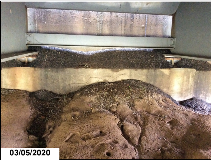
debris at end bents
