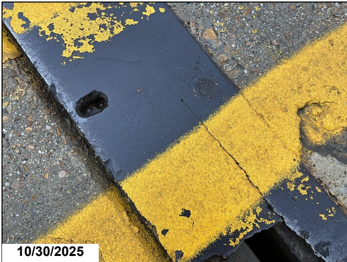
Bent 3, Joint. Cracking in the joint armor. 1LF CS3 metal deterioration.
