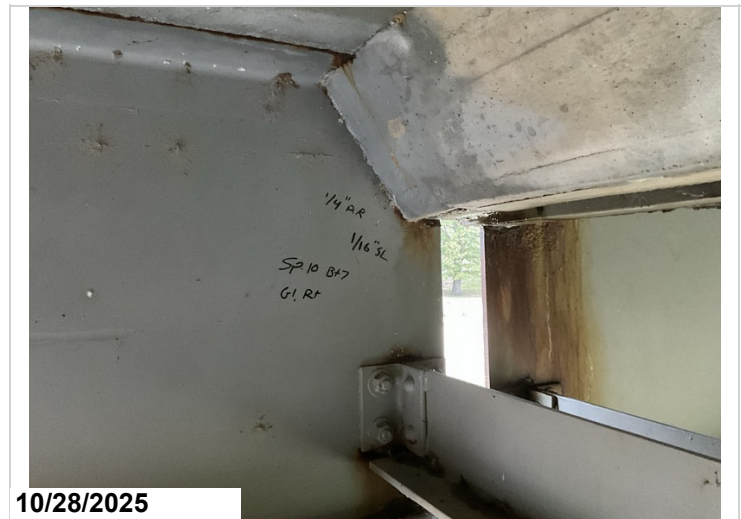
Span 10, Bent 7, Girder 1, Right: Active corrosion with section loss up to 1/16" to the web at the haunch area and pack rust up to 1/4" between the girder web and the concrete haunch. 1LF CS3 corrosion.
