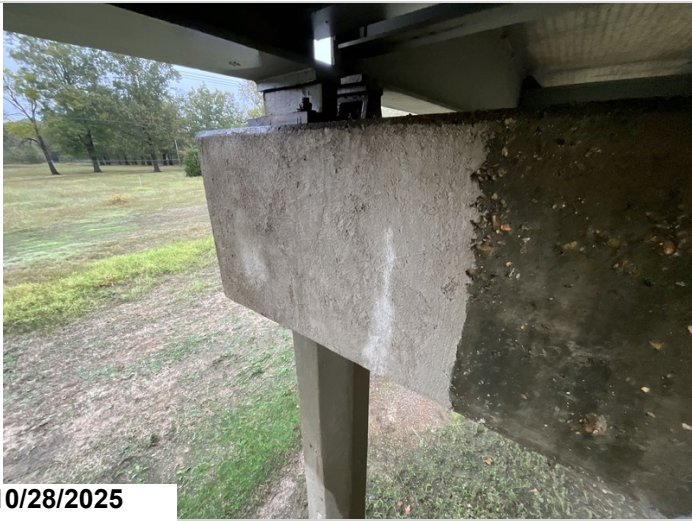
Bent 3, Back, under Girder 1: Repair. 4LF CS2 patch.
