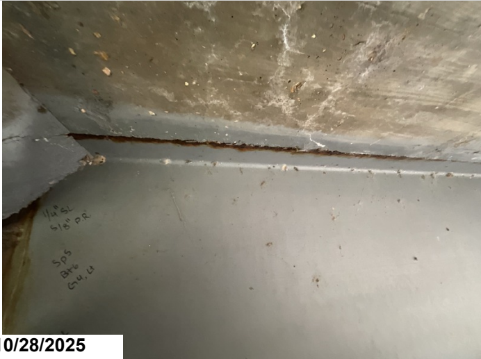
Span 5, Girder 4, Left: Active corrosion with flaking rust along the Top Flange. 5LF CS3 corrosion.
