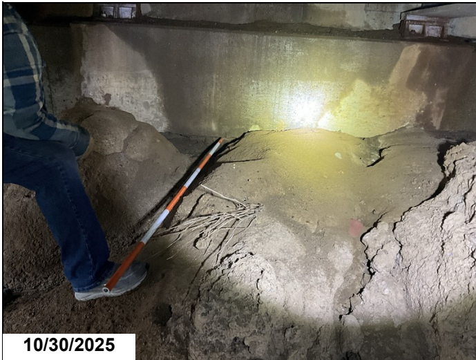
Bent 8: Erosion along the bottom of the bridge seat with undermining up to 1.5'. 18LF CS2 Scour.
