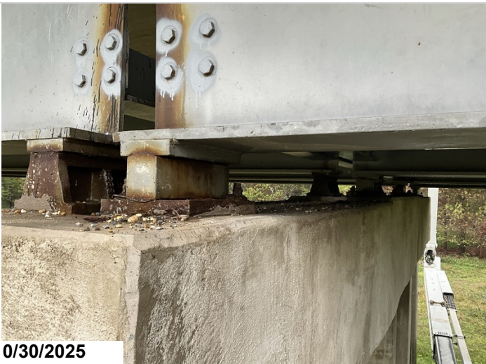
Span 1, Bent 2, Bearings: Active corrosion with pack rust. 4EA CS3 corrosion.
