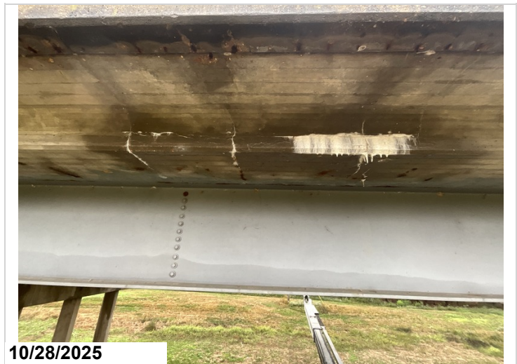
Span 3, Left overhang: Cracking with efflorescence build up and rust staining. 25sf CS3 efflorescence/rust staining.
