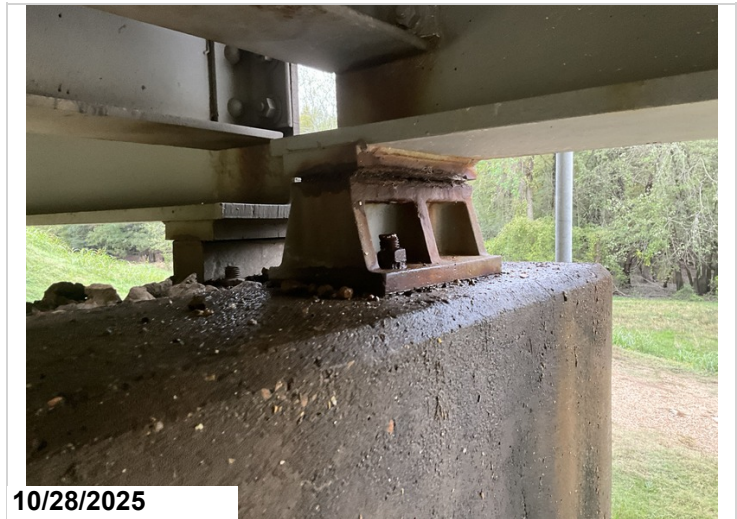
Span 10, Bent 7, Bearings 1 - 4: Active corrosion with pack rust. 4EA CS3 corrosion.
