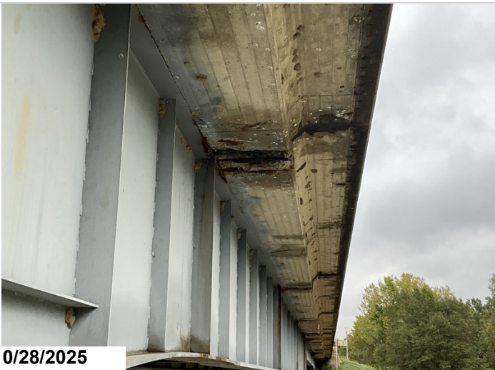
Span 9, Right overhang: Spalling with exposed reinforcing steel with section loss. 19sf CS3 corrosion.
