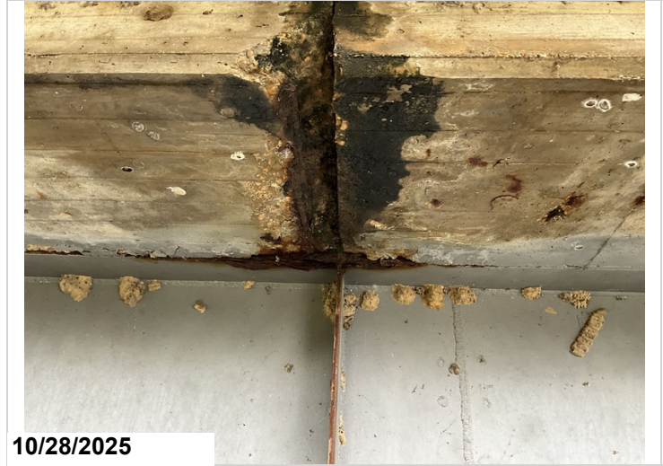
Span 9, Girder 1, Left: Active corrosion with flaking rust along the Top Flange below first saw joint.
