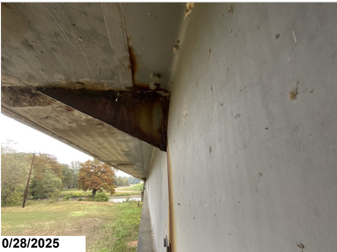
Span 3, Bent 4, Girder 1: Minor distortion in web due to pack rust between the Girder web and concrete haunch.
