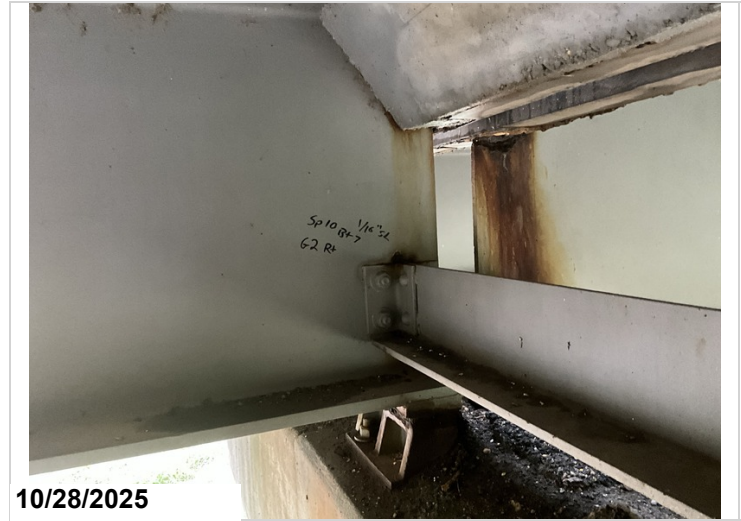
Span 10, Bent 7, Girder 2, Right: Active corrosion with section loss up to 1/16" to the web at the diaphragm connection. 1LF CS3 corrosion.
