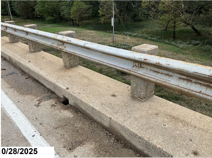
Span 2: Cracked bridge railing post.
