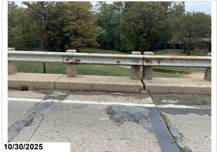
Span 10, Left: Active corrosion to the railing.
