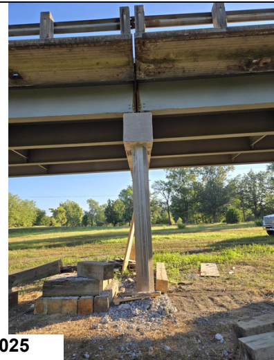
Bent 3 Cap: Repaired
