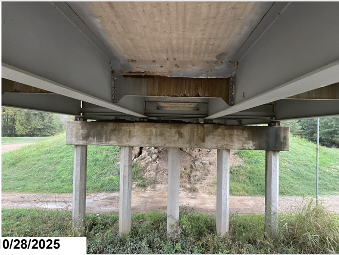
Bent 7, Cap: Needs cleaned.
