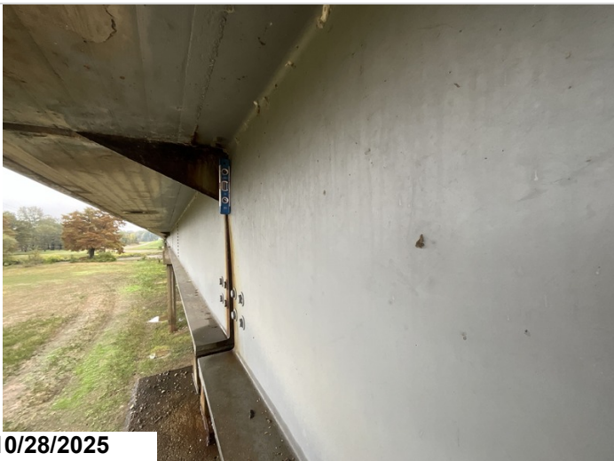
Span 2, Bent 3, Girder 1, Left: Minor distortion in the web due to pack rust between Girder web and concrete haunch.
