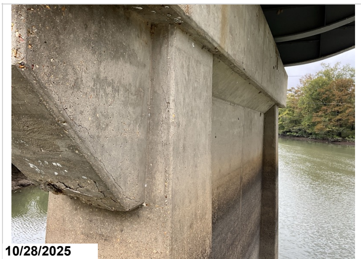
Pier 2, Column 2, Right: Vertical cracking. 1EA CS2 cracking.
