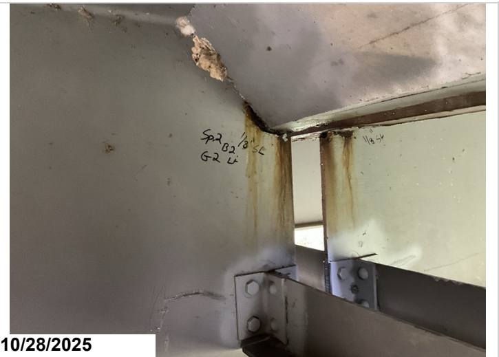
Span 2, Bent 2, Girder 2, Left: Active corrosion with section loss up to 1/8" section loss to the web in the haunch area. 1LF CS3 corrosion.
