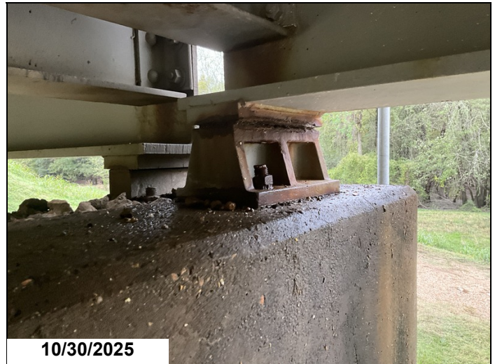
Span 10, Bent 7, Bearings 1 - 4: Active corrosion with pack rust. 4EA CS3 corrosion.
