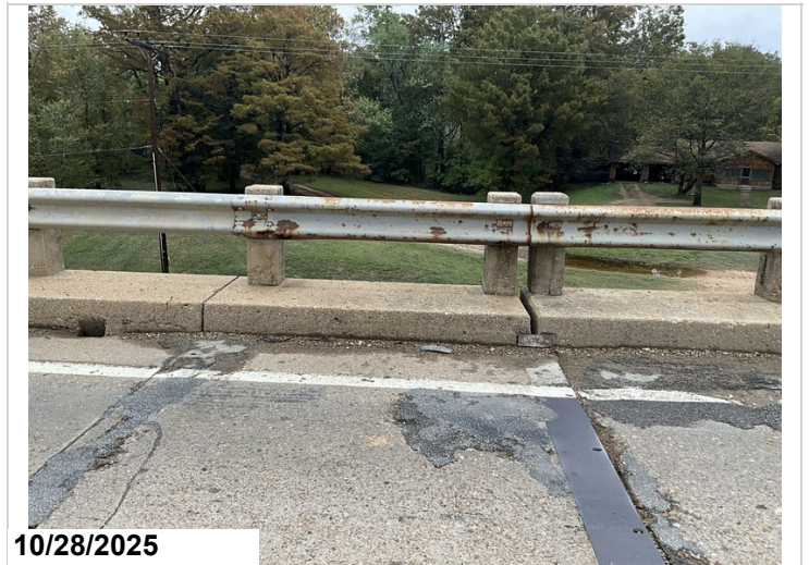
Span 10, Left: Active corrosion to the railing.
