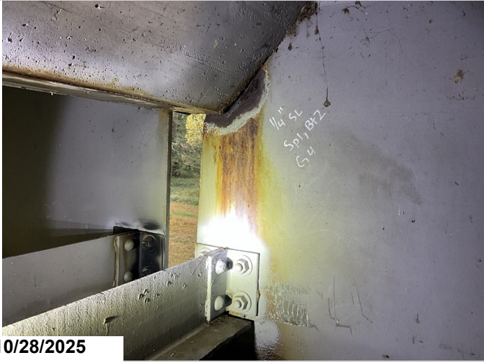
Span 1, Bent 2, Girder 4: Active corrosion with section loss up to 1/4" to the web at the haunch area. 1LF CS3 corrosion
