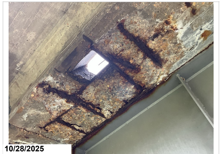
Span 7, Right overhang: Spalling with exposed reinforcing steel with section loss. 18SF CS3 exposed reinforcing steel.
