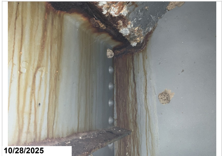
Span 6, Girders 1 - 4, at center Two diaphragms: Active corrosion with with flaking rust and section loss up to 3/16" to the web at the haunch areas. 8LF CS3 corrosion.
