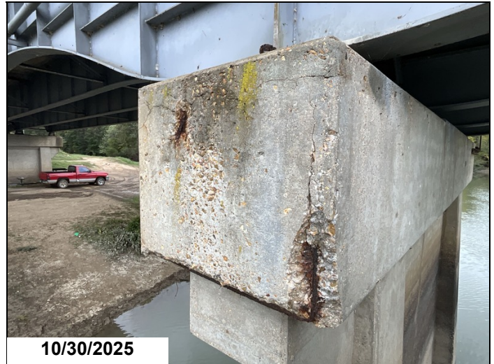
Pier 3, Cap, Left: Spalling with exposed reinforcing steel with section loss. 1LF CS3 exposed reinforcing steel.
