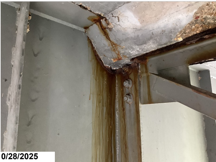
Span 6, Pier 1, Girders: Typical Active corrosion with flaking rust to the web at the concrete haunch areas.
