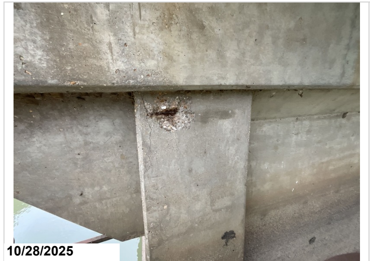
Pier 3, Column 2, Ahead: Spalling with exposed reinforcing steel with section loss near bottom of cap. 1EA CS3 exposed reinforcing steel.
