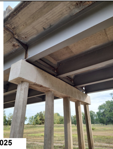
Bent 4, Cap: Repaired
