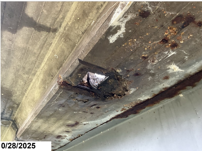
Span 6, Left overhang: Spalling with exposed reinforcing steel with section loss. 11SF CS3 exposed reinforcing steel.
