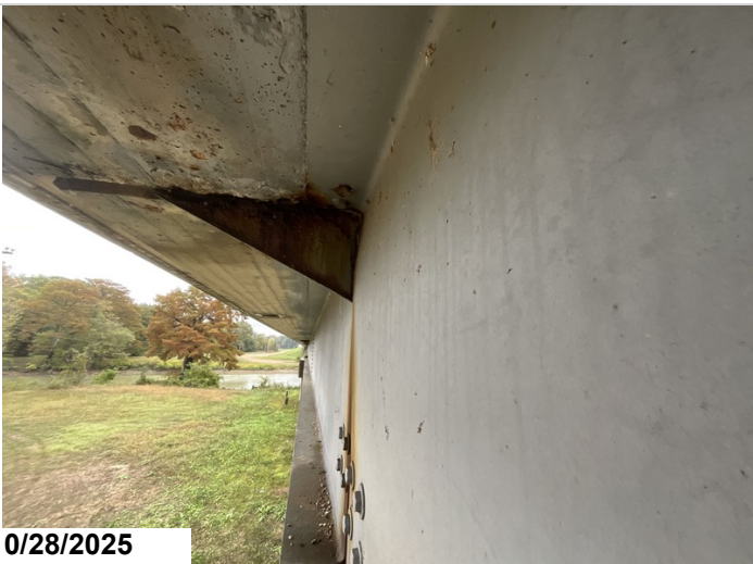
Span 4, Bent 5, Girder 1: Minor distortion in the web due to pack rust between the Girder web and concrete haunch.
