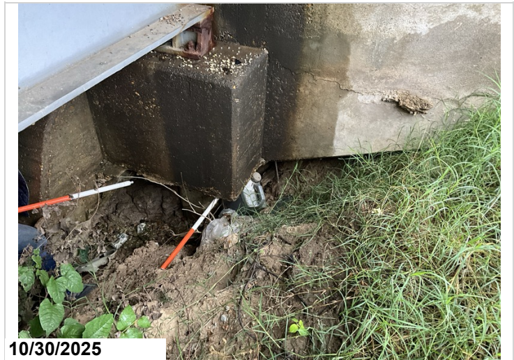
Bent 1: Erosion up to 2' below the bottom of the bridge seat under Girders 1 and 4, worst being under Girder 1 with undermining up to 2.5'. 6LF CS2 erosion, 10LF CS3 erosion.
