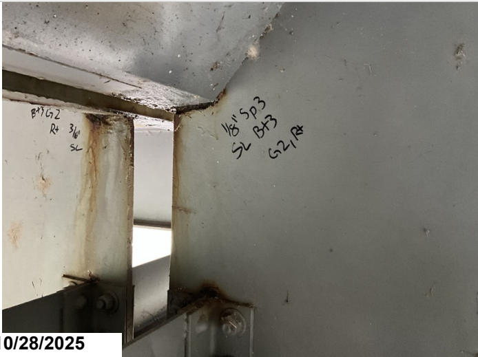
Span 3, Bent 3, Girder 2, Right: Active corrosion with section loss up to 1/8" to the web at the haunch area. 1LF CS3 corrosion.
