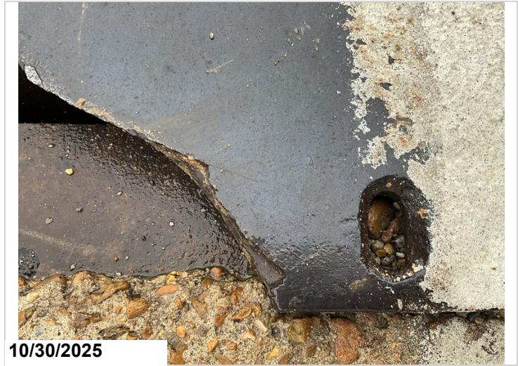
Bent 6, Joint: Cracking in the joint armor. 1LF CS3. metal deterioration.
