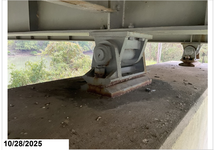
Pier 1: Typical bearings.
