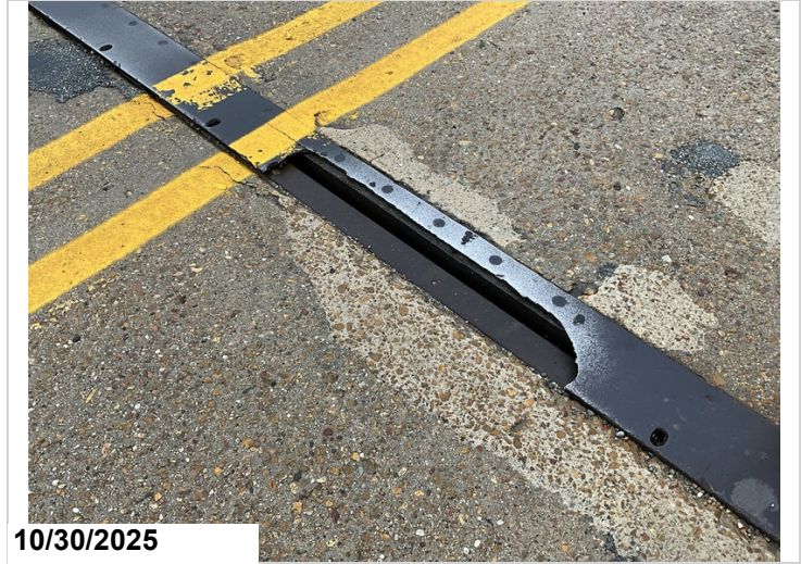
Bent 3, Joint: Armor missing. 4LF CS4 metal deterioration.
