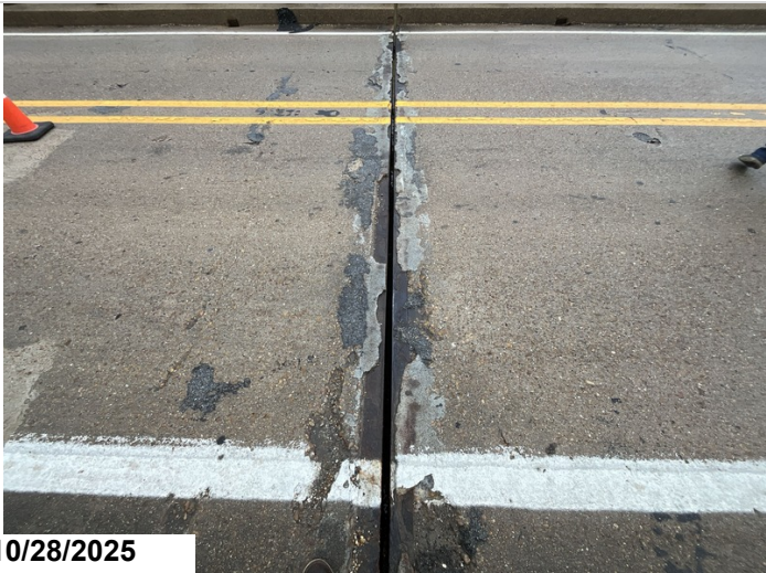
Bent 5, Joint: Armor missing for the full length. 26LF CS4 metal deterioration.
