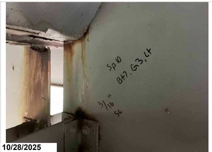
Span 10, Bent 7, Girder 3, Left: Active corrosion with section loss up to 3/16" to the web at the diaphragm connection. 1LF CS3 corrosion.
