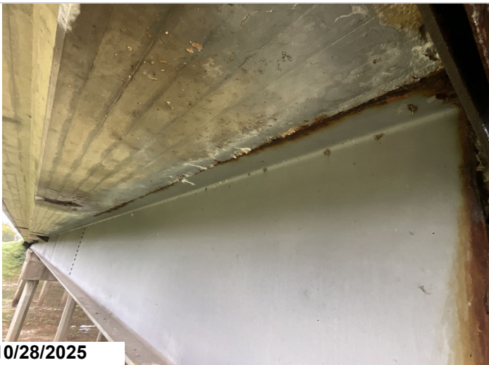
Span 5, Girder 4, Right: Active corrosion with flaking rust along the Top Flange. 18LF CS3 corrosion.
