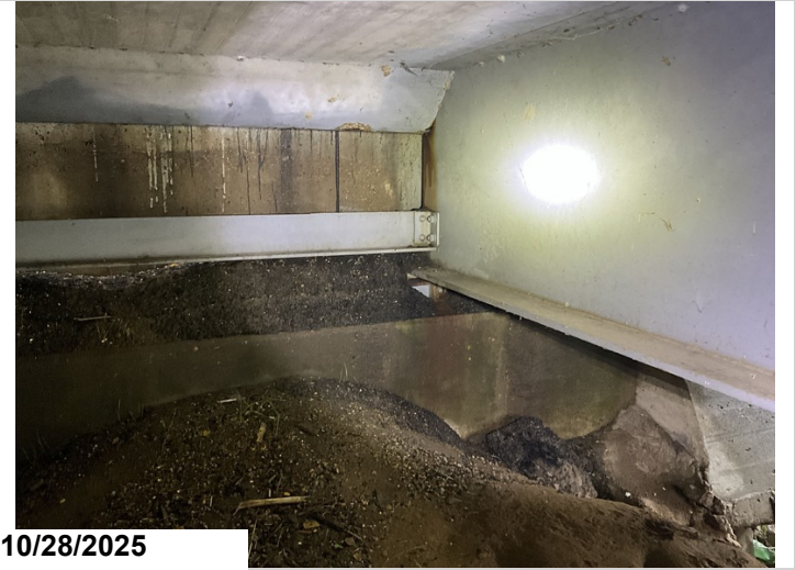
Span 1, Bent 1, Girders 1 - 4: Active corrosion with flaking rust to the web in the haunch areas. 4LF CS3 corrosion.
