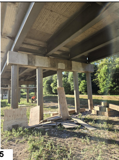
Bent 3 Cap: Repaired
