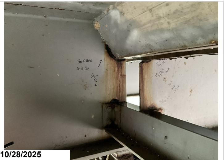
Span 6, Bent 6, Girder 3, Left: Active corrosion with section loss up to 1/4" to the web at the haunch and diaphragm connection areas. 1LF CS3 corrosion.
