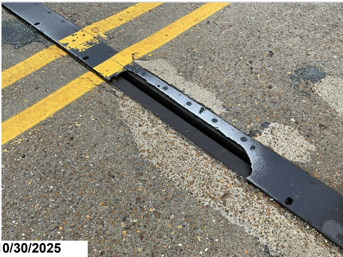
Bent 3, Joint: Armor missing. 4LF CS4 metal deterioration.
