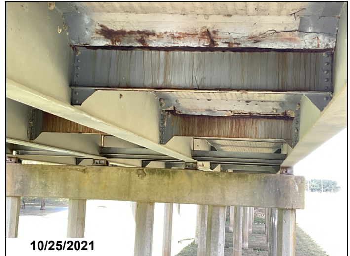
Span 6 diaphragms
