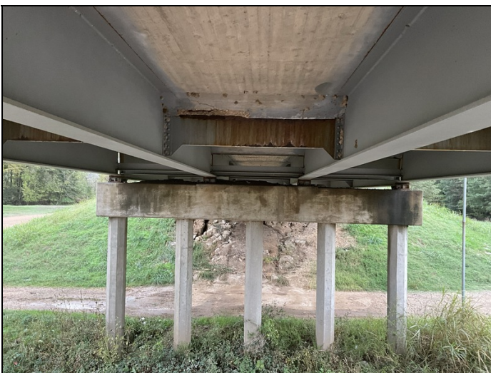
Bent 7, Cap: Needs cleaned.
