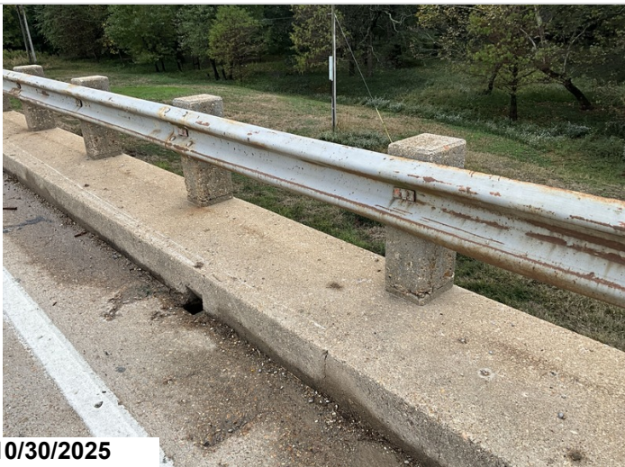
Span 2: Cracked bridge railing post.
