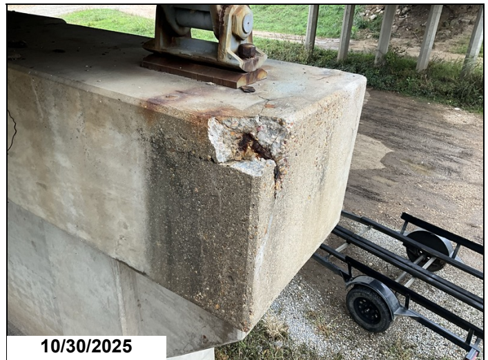
Pier 4, Right, back corner: Spalling with exposed reinforcing steel with section loss. 1LF CS3 exposed reinforcing steel.
