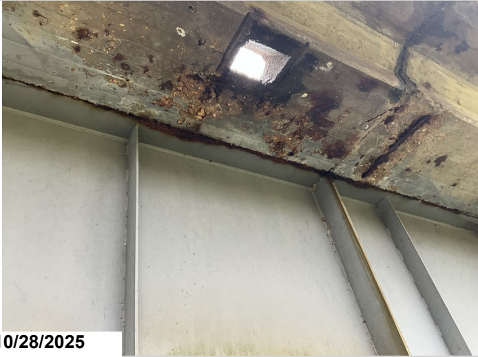
Span 7, Girder 1, Left: Active corrosion with flaking rust along the Top Flange. 22LF CS3 corrosion.
