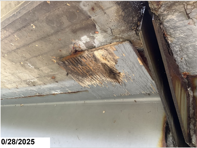
Span 3, Right overhang, near Bent 4: Patched area. 2SF CS3 unsound patch.
