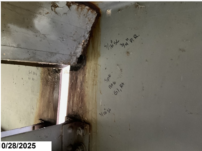
Span 6, Bent 6, Girder 1, Right: Active corrosion with section loss up to 5/16" to the web at the haunch area, section loss up to 3/16" to the web at the diaphragm connection, and pack rust up to 3/4" between the girder web and the concrete haunch. 1LF CS3 corrosion.
