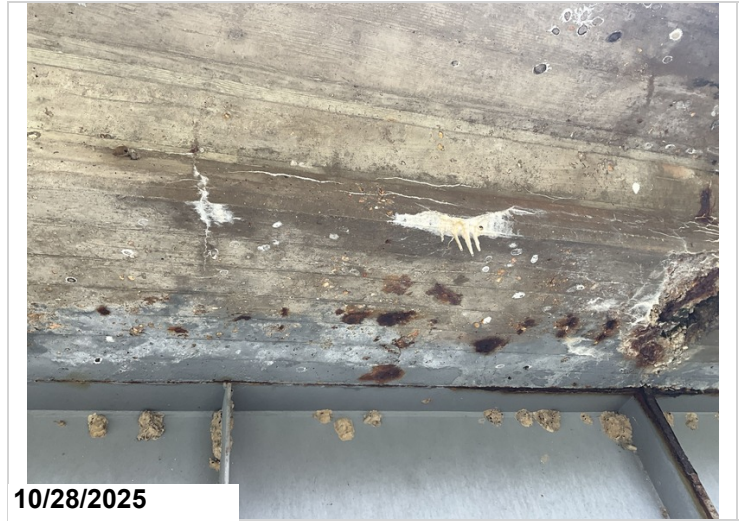
Span 8, Left overhang: Cracking with efflorescence build up. 8SF CS3 efflorescence.
