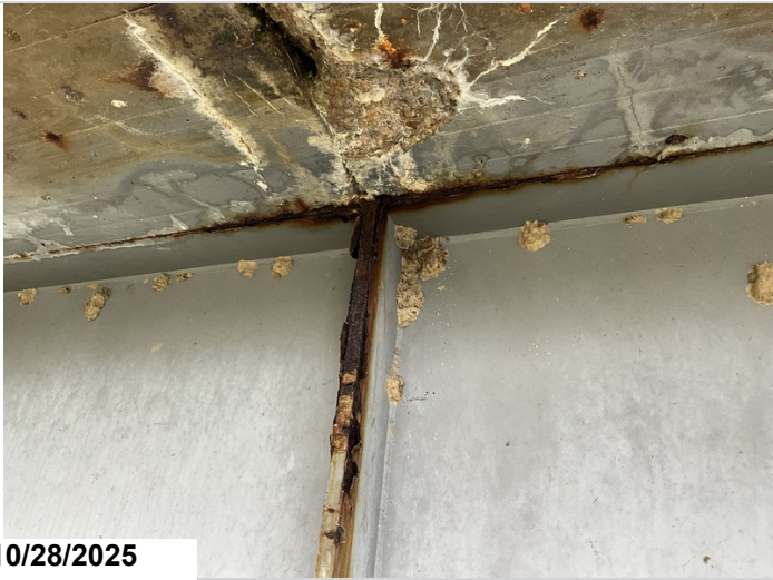
Span 8, Pier 3, Girder 1, Left: Active corrosion with flaking rust along the Top Flange and vertical bearing stiffener. 4LF CS3 corrosion.
