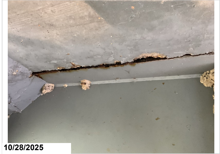
Span 7, Girder 2, Right: Active corrosion with flaking rust along the Top Flange. 7LF CS3 corrosion.
