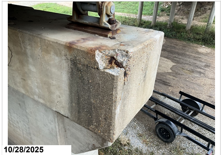
Pier 4, Right, back corner: Spalling with exposed reinforcing steel with section loss. 1LF CS3 exposed reinforcing steel.
