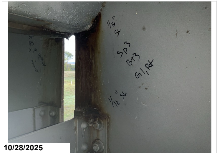
Span 3, Bent 3, Girder 1, Right: Active corrosion with section loss up to 1/16" to the web at the haunch and diaphragm connection areas. 1LF CS3 corrosion.
