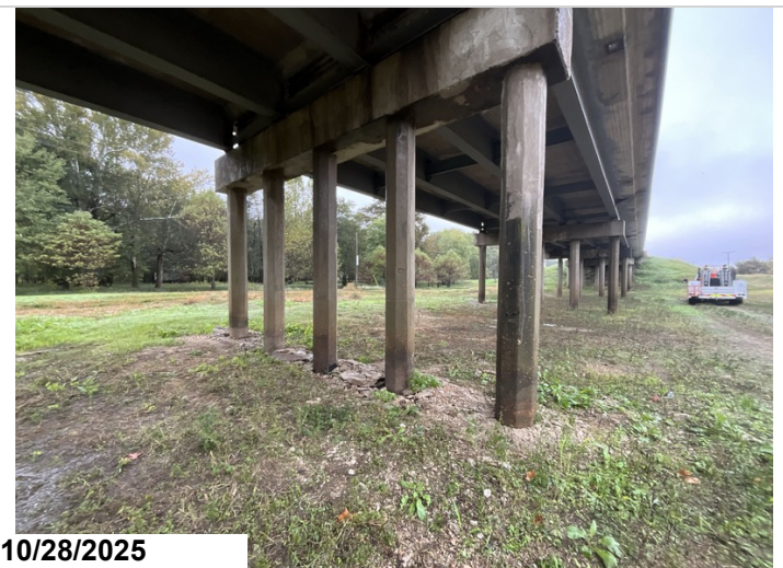
Bent 5, Piles 1 - 5: Minor abrasion. 5EA CS2 abrasion.
