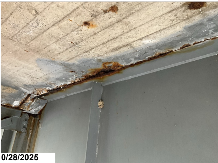
Span 9, back of Pier 4, Girder 4, Left: Active corrosion with flaking rust along the Top Flange. 12LF CS3 corrosion.
