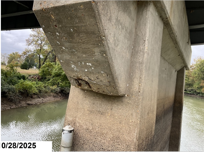
Pier 2, Right, Bottom cap: Spalling with exposed reinforcing steel with section loss. 1LF CS3 corrosion.
