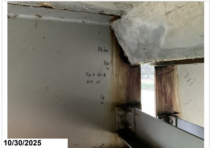
This defect is common throughout the structure at girder ends.
