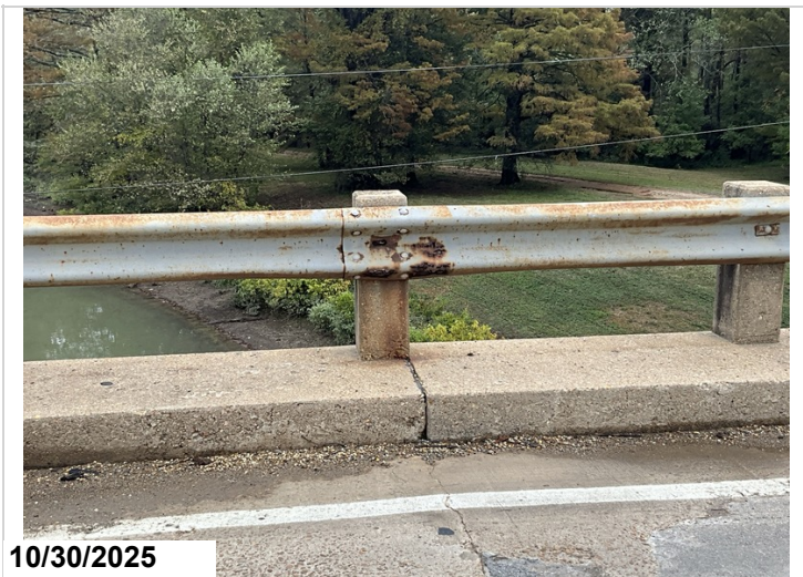
Span 8, Left, Last post: Missing bolt from railing to post.
