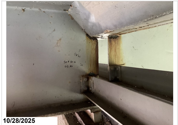
Span 5, Bent 6, Girder 3, Right: Active corrosion with section loss up to 1/8" to the web at the haunch and diaphragm connection areas. 1LF CS3 corrosion.
