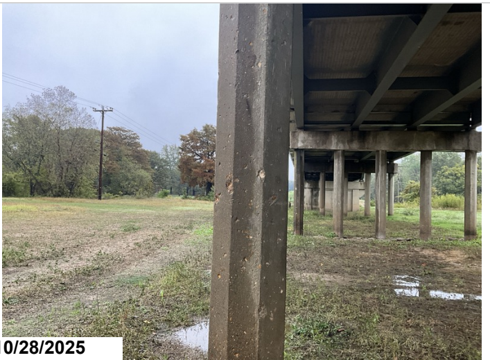
Bent 4, Pile 1: Minor spalling on the back side. 1EA CS2 Spalling.
