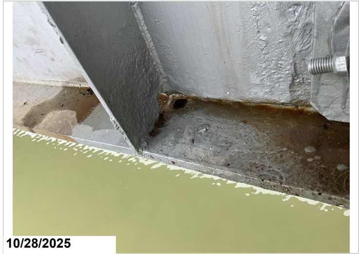
Span 8, Girder 4, Right, Last stiffener before second Pin and Hanger Assembly: Hole in vertical Stiffener.
