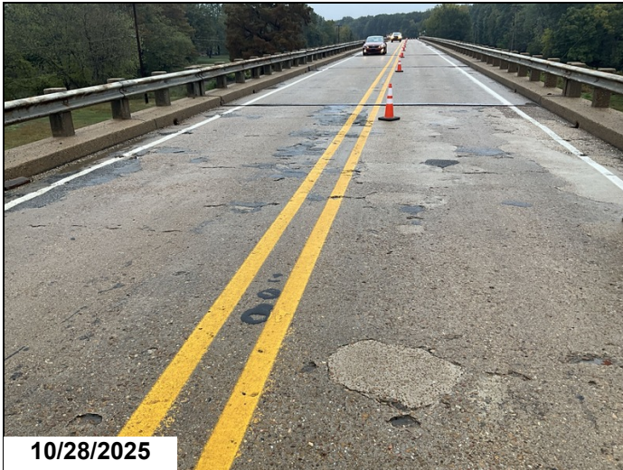
Span 3: Unsound patches, sound patches, cracking, abrasion, and spalling.
