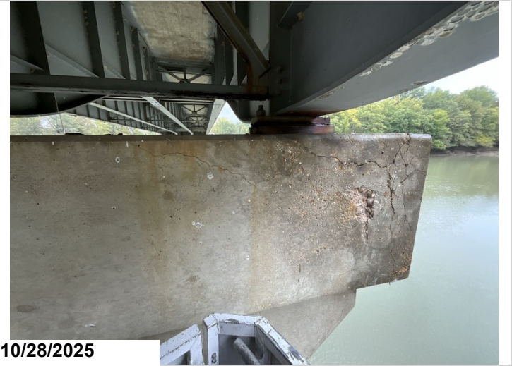
Pier 2, Cap, Back: Cracking and spalling under Girder 4. 5LF CS3 cracking and 1LF CS3 spalling.
