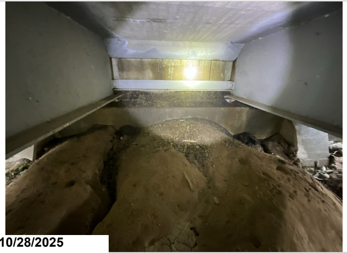
Bent 1: Cap needs cleaned.
