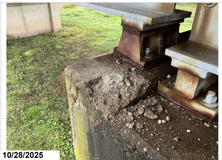
Bent 6, Left: Spalling with exposed reinforcing steel with section loss. 1LF CS3 exposed reinforcing steel.
