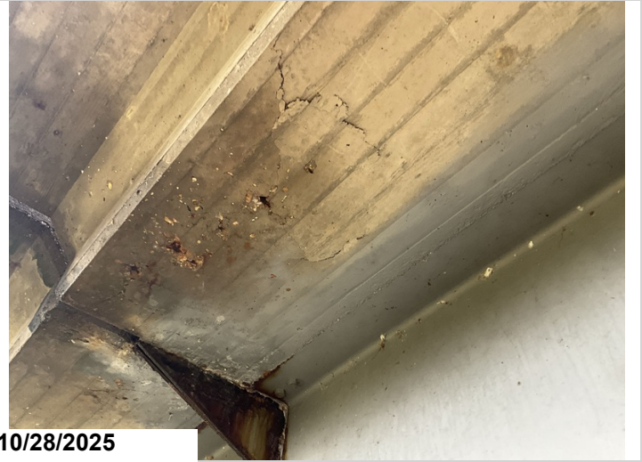
Span 2, Left overhang, Adjacent to Bent 3: Delamination area. 2SF CS2 delam.
