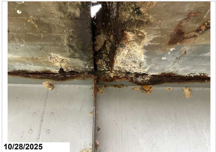
Span 7, Girder 1, Left, Top Flange: Active corrosion with flaking rust along the Top Flange below last saw joint before Pier 2. 8LF CS3 corrosion.
