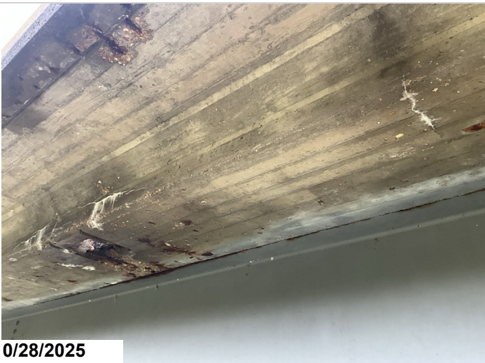
Span 4, Right overhang: Cracking with efflorescence build. 5SF CS3 efflorescence.
