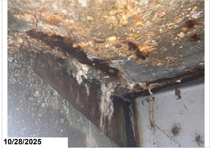
Span 11, Left overhang, Adjacent to Bent 8: Spalling with exposed reinforcing steel with section loss. 2SF CS3 exposed reinforcing steel.
