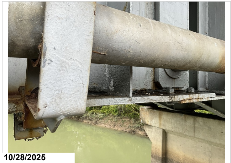
Span 8, Girder 1, First stiffener after first Pin and Hanger Assembly: Hole in vertical stiffener.
