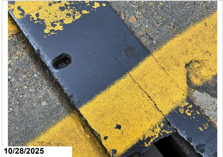
Bent 3, Joint. Cracking in the joint armor. 1LF CS3 metal deterioration.
