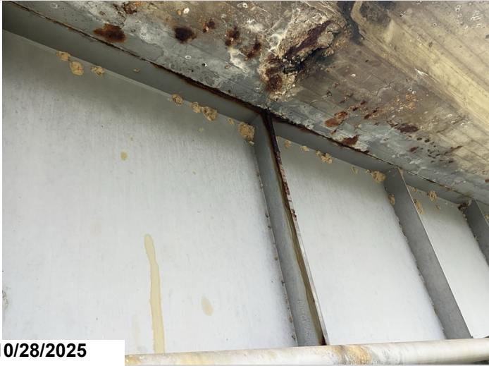
Span 8, Girder 1, Left: Active corrosion with flaking rust along the Top Flange and vertical bearing Stiffener. 6LF CS3 corrosion.
