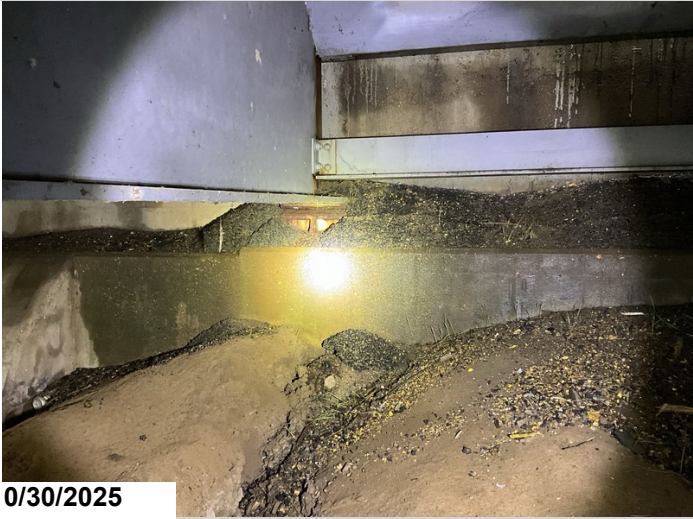
Bent 1, Bearings 1 - 4: Active corrosion with pack rust. 4EA CS3 corrosion.
