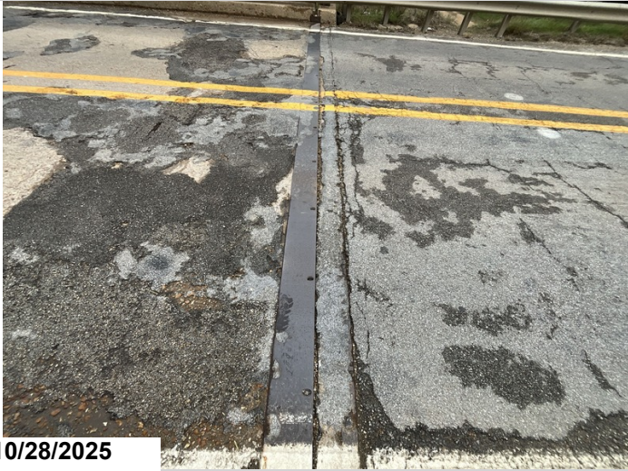
Bent 8, Joint: Debris impact, full length. 26LF CS3 debris impact.
