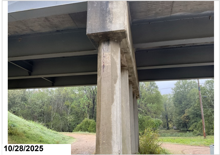
Bent 7, Pile 1, Ahead and Left: Vertical cracking with rust staining. 1EA CS3 rust staining.
