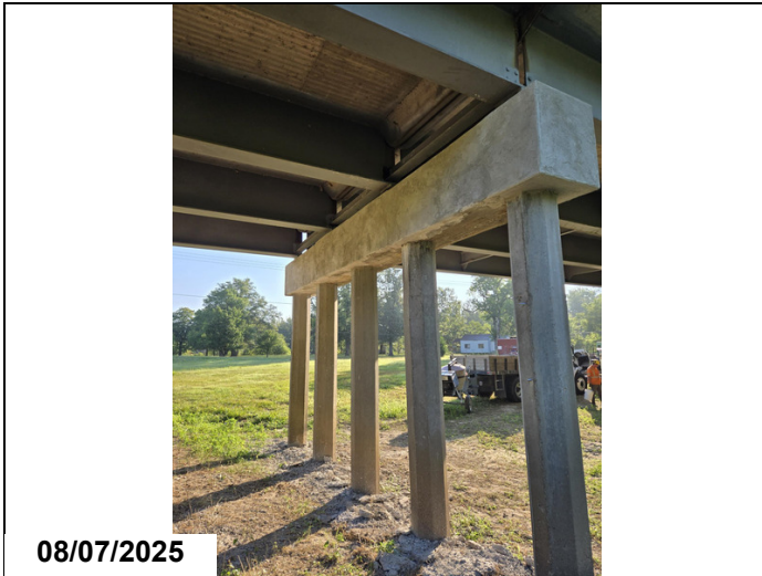
Bent 2 Cap: Repaired w/Galvanic Anodes
