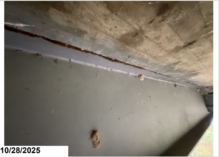
Span 6, Girder 1, Right, Top Flange: Active corrosion with flaking rust along the Top Flange. 12LF CS3 corrosion. Left side mirrors.
