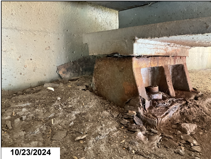
Bent 8, bearing 3: floating bearing.
