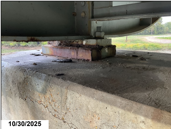
Pier 2, Bearings 1 - 4: Active corrosion with pack rust between the sole and masonry plate. 4EA CS3 corrosion.
