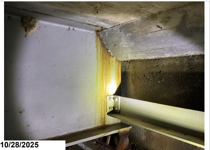
Span 11, Bent 8, Girder 1: Active corrosion with flaking rust. 1LF CS3 corrosion.
