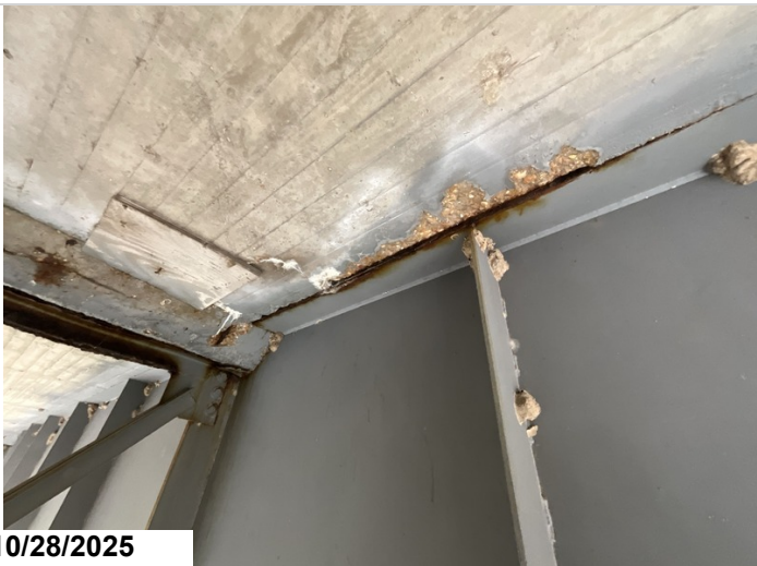
Span 8, Girder 3, Right: Active corrosion with flaking rust along the Top Flange. 11LF CS3 corrosion.
