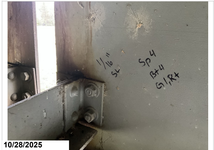
Span 4, Bent 4, Girder 1, Right: Active corrosion with section loss up to 1/16" to the web at the diaphragm connection. 1LF CS3 corrosion.
