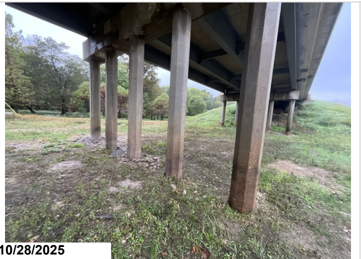
Bent 3, Piles 1 - 5: Minor abrasion. 5EA CS2 abrasion.
