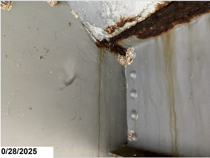
Span 6, Girders 1 - 4, at center Two diaphragms: Active corrosion with with flaking rust and section loss up to 3/16" to the web at the haunch areas. 8LF CS3 corrosion.
