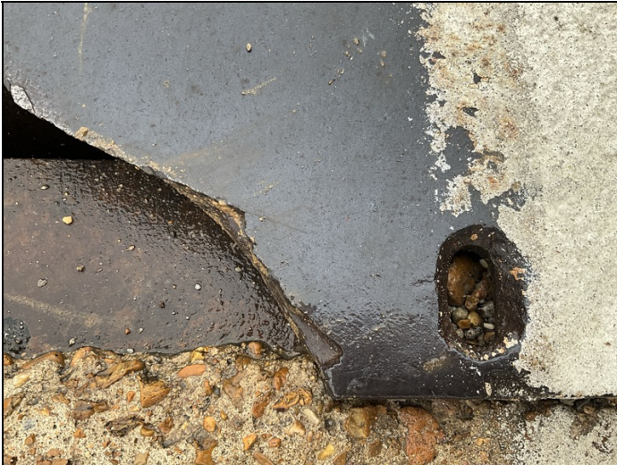
Bent 6, Joint: Cracking in the joint armor. 1LF CS3. metal deterioration.
