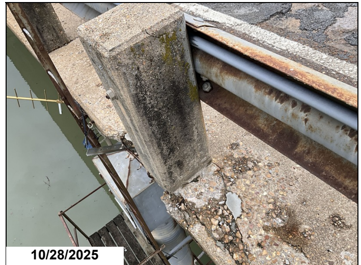
Span 9, Right: Spalling at bridge railing post.
