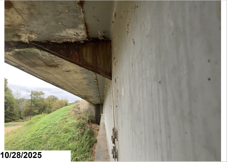
Span 10, Bent 7, Girder 1: Distortion in the web due to pack rust between the Girder web and concrete haunch.
