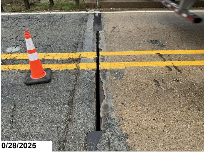
Bent 1, Joint: Armor missing. 12LF CS4 metal deterioration.
