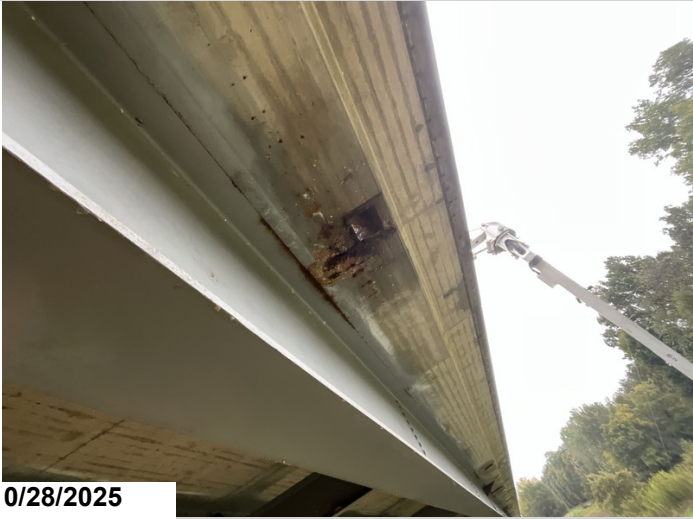
Span 5, Right overhang: Spalling with exposed reinforcing steel with section loss at the drain locations. 2SF CS3 exposed reinforcing steel.
