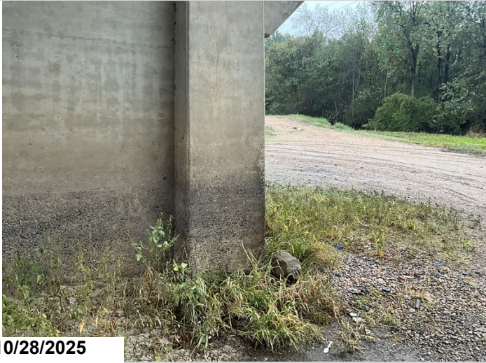
Pier 4, Column 2: Abrasion. 1EA CS2 abrasion.
