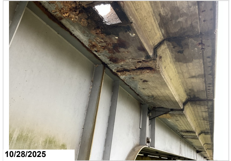
Span 7, Left overhang: Spalling with exposed reinforcing steel with section loss. 8SF CS3 exposed reinforcing steel.
