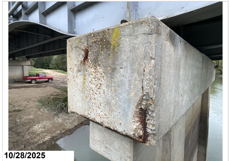
Pier 3, Cap, Left: Spalling with exposed reinforcing steel with section loss. 1LF CS3 exposed reinforcing steel.
