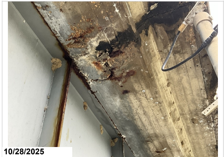
Span 9, Right overhang: Spalling with exposed reinforcing steel with section loss. 19sf CS3 corrosion.
