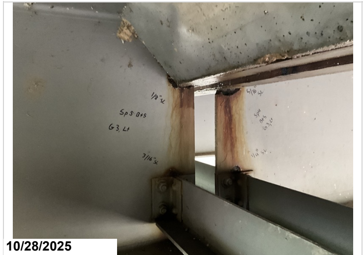
Span 5, Bent 5, Girder 3, Left: Active corrosion with section loss up to 1/8" to the web at the haunch area and section loss up to 3/16" to the web at the diaphragm connection. 1LF CS3 corrosion.
