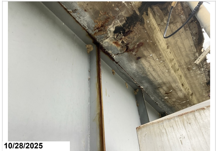
Span 8, Girder 4, Right: Active corrosion with flaking rust along the Top Flange and vertical bearing stiffener. 4LF CS3 corrosion.
