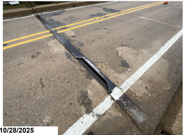
Bent 6, Joint: Joint armor missing. 4LF CS4 metal deterioration.
