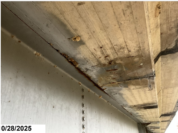
Span 10, Girder 1, Left: Active corrosion with flaking rust along the Top Flange. 7LF CS3 corrosion.
