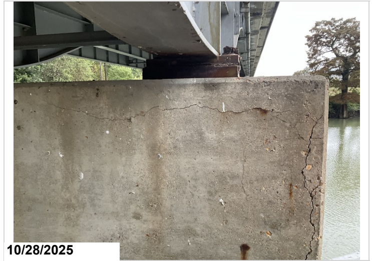
Pier 3, Ahead, Cap, below Girder 1: Horizontal cracking. 4LF CS3 cracking.
