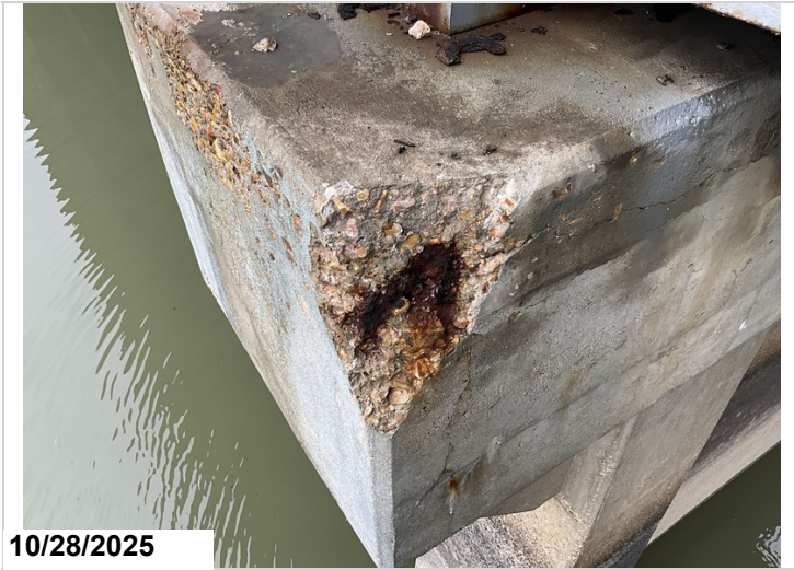
Pier 2, Back, Left corner: Spalling with exposed reinforcing steel with section loss. 1LF CS3 exposed reinforcing steel.
