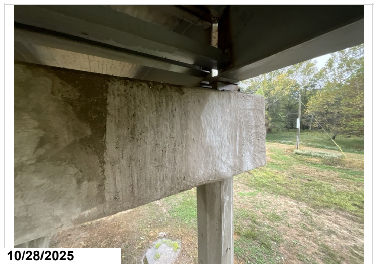
Bent 3, back, under Girder 4: Repair. 4LF CS2.
