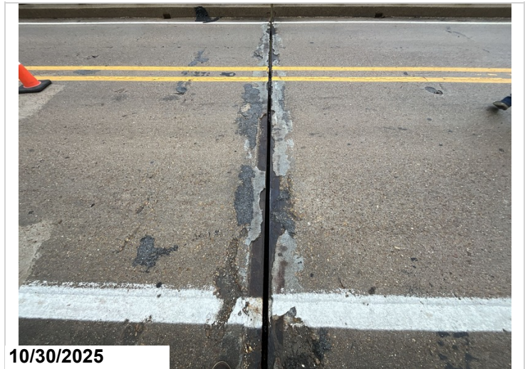
Bent 5, Joint: Armor missing for the full length. 26LF CS4 metal deterioration.
