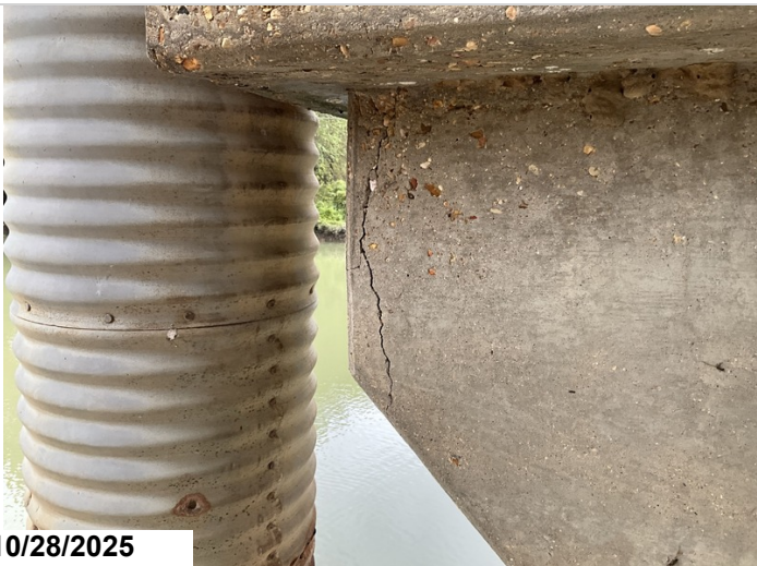
Pier 3, Right, Bottom: 1LF CS3 vertical cracking.
