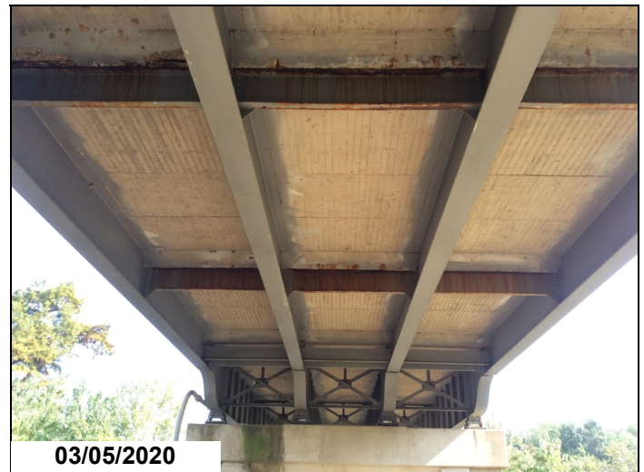
Span 6 leakage thru deck onto diaphragms
