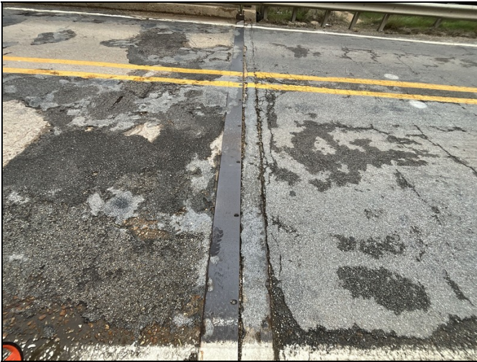
Bent 8, Joint: Debris impactation, full length. 26LF CS3 debris impactation.
