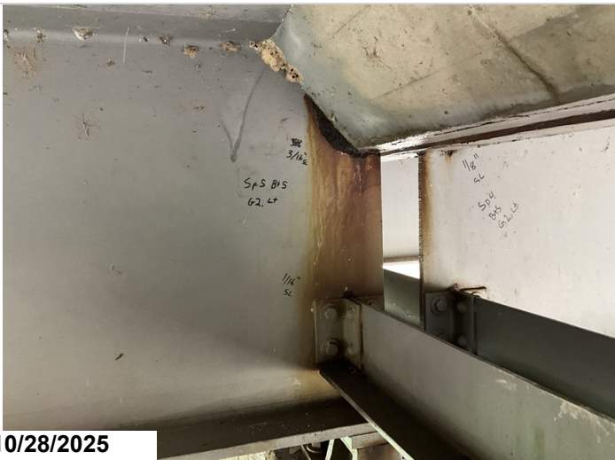
Span 5, Bent 5, Girder 2, Left: Active corrosion with section loss up to 3/16" to the web at the haunch area and section loss up to 1/16" to the web at the diaphragm connection. 1LF CS3 corrosion.
