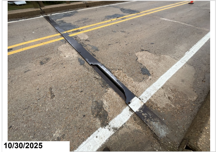
Bent 6, Joint: Joint armor missing. 4LF CS4 metal deterioration.
