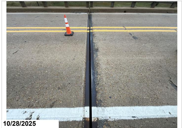
Bent 2, Joint: Armor missing for the full length. 26LF CS4 metal deterioration.
