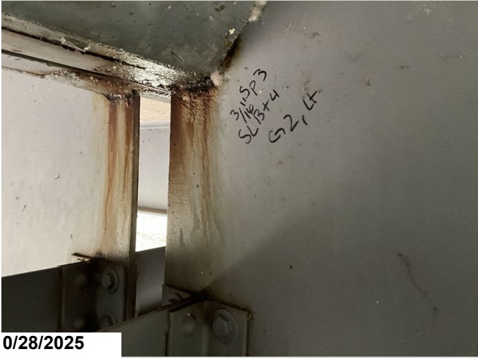
Span 3, Bent 4, Girder 2, Left: Active corrosion with section loss up to 3/16" to the web at the haunch area. 1LF CS3 corrosion.
