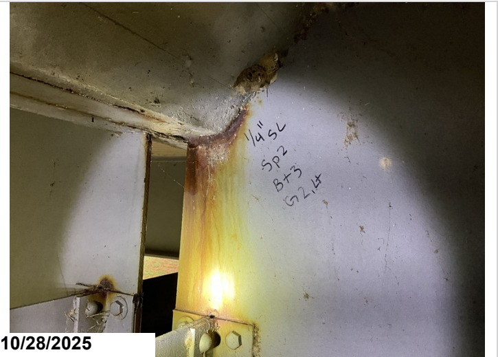
Span 2, Bent 3, Girder 2, Left: Active corrosion with section loss up to 1/4" to the web at haunch area. 1LF CS3 corrosion.
