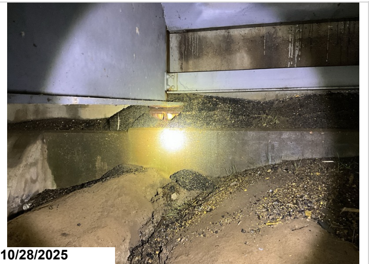
Bent 1, Bearings 1 - 4: Active corrosion with pack rust. 4EA CS3 corrosion.
