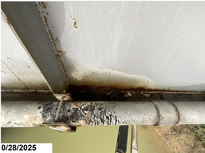
Span 7, Girder 1, Left, Web: Active corrosion with laminated rust build up below last saw joint before Pier 2.
