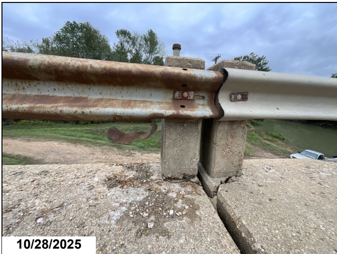
Span 11, Right: Damage to bridge railing. 2LF CS3 damage.
