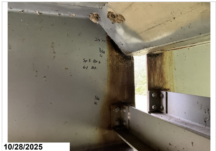
Span 5, Bent 6, Girder 1, Right: Active corrosion with section loss up to 3/16" to the web at the haunch area, section loss up to 1/16" to the web at the diaphragm connection, and pack rust up to 3/4" between the girder web and the concrete haunch. 1LF CS3 corrosion.
