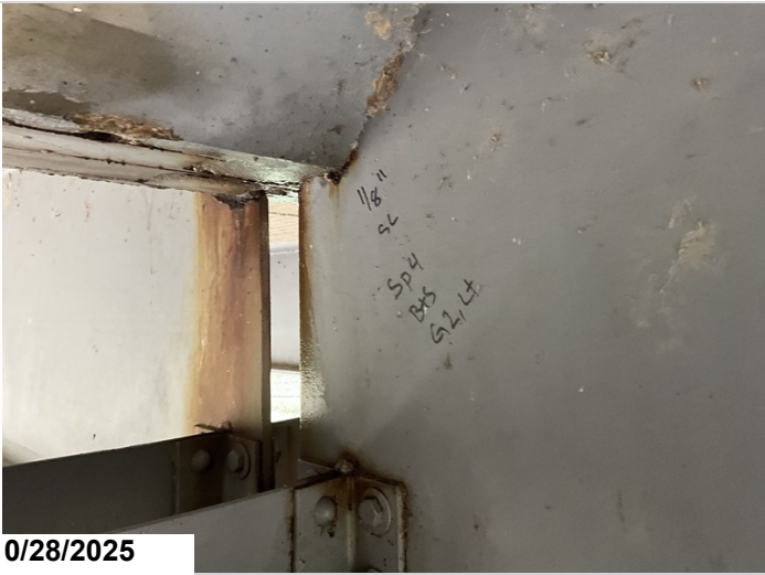
Span 4, Bent 5, Girder 2, Left: Active corrosion with section loss up to 1/8" to the web at the haunch area. 1LF CS3 corrosion.
