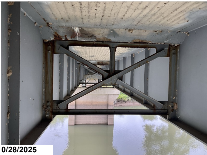
Span 8: Typical corrosion around diaphragms.
