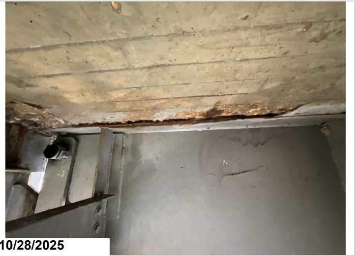
Span 6, Girder 1, Right, Between Pin and Hanger Assembly and Pier 1: Active corrosion with flaking rust along the Top Flange. 5LF CS3 corrosion.
