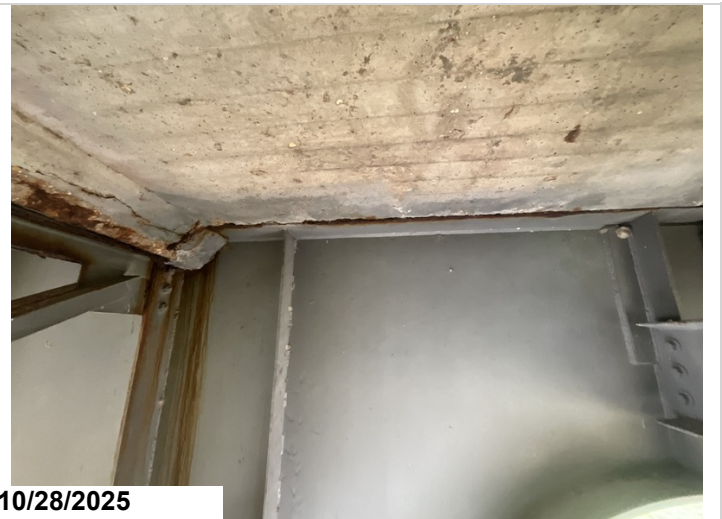
Span 6, Girder 4, Left. Between Pin and Hanger Assembly and Pier 1: Active corrosion with flaking rust along the Top Flange. 8LF CS3 corrosion.
