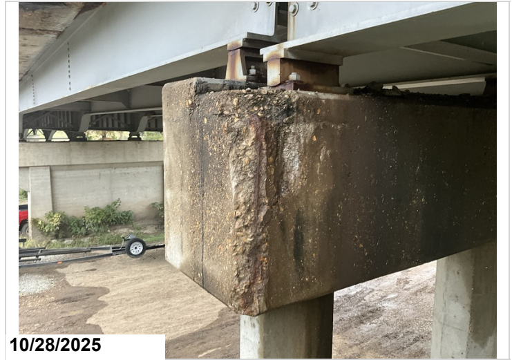
Bent 7, Ahead, Right: Spalling with exposed reinforcing steel with section loss. 1LF CS3 exposed reinforcing steel.
