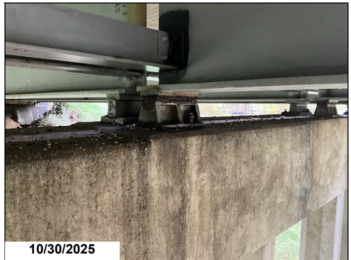
Span 2, Bent 2, Bearings: Active corrosion with pack rust up to 1" between bearing and sole plate. 4ea CS3 corrosion.
