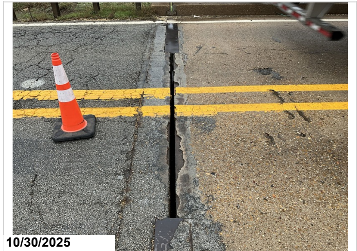
Bent 1, Joint: Armor missing. 12LF CS4 metal deterioration.
