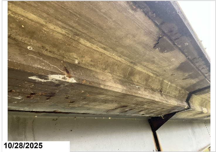
Span 6, Left overhang: Cracking with efflorescence and rust staining. 8SF CS3 efflorescence/rust staining.
