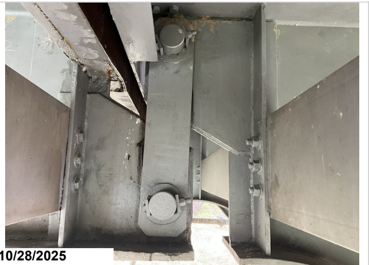
Span 6, Pin and Hanger Assemblies: Replaced since last inspection.
