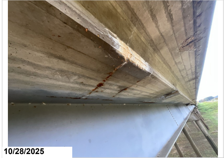
Span 5, Left overhang: Cracking with efflorescence and rust staining. 3LF CS3 efflorescence/rust staining.
