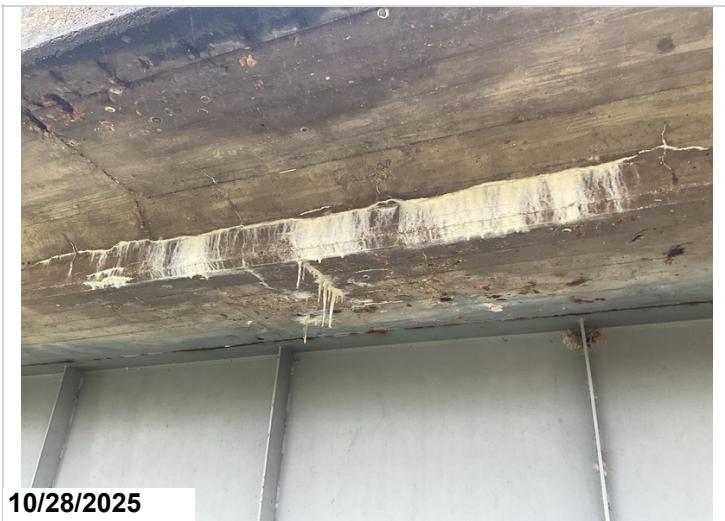
Span 7, Left overhang: Cracking with efflorescence. 18SF CS3 efflorescence.
