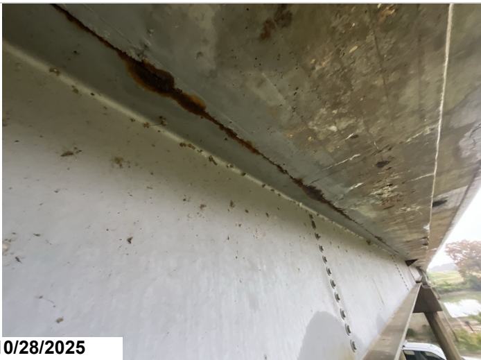
Span 11, Girders 1 - 4: Active corrosion with flaking rust along the Top Flange. 115LF CS3 corrosion.
