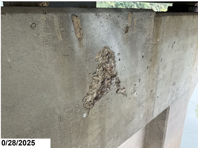
Pier 2, Cap, Back: Spalling below Girder 3. 2LF CS3 spalling.
