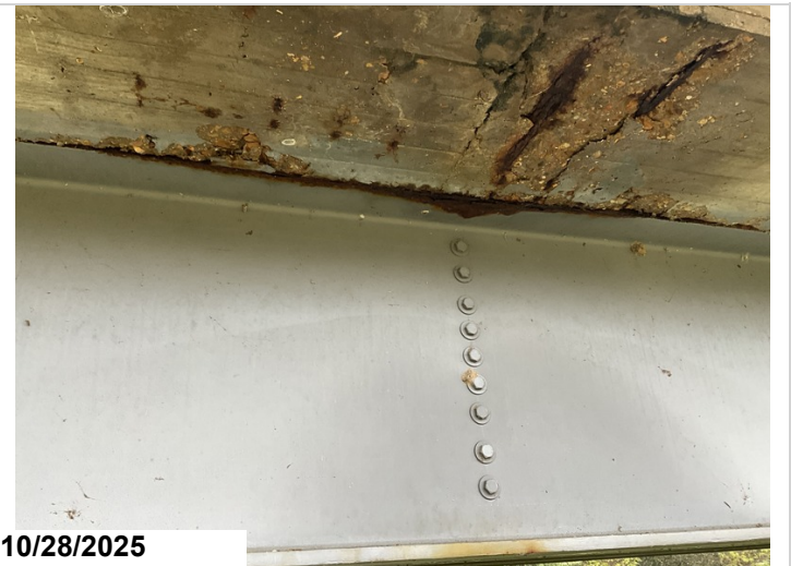
Span 6, Girder 1, Left: Active corrosion with flaking rust along the Top Flange. 7LF CS3 corrosion.
