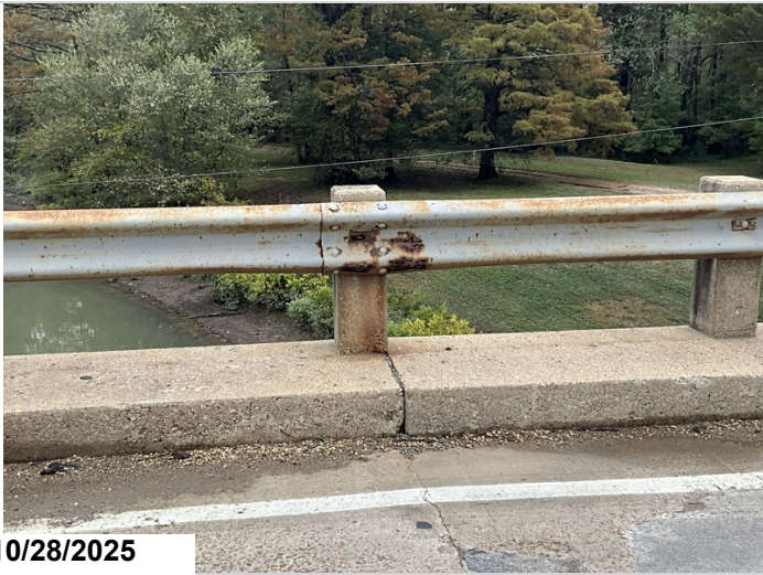
Span 8, Left, Last post: Missing bolt from railing to post.
