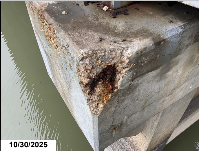
Pier 2, Back, Left corner: Spalling with exposed reinforcing steel with section loss. 1LF CS3 exposed reinforcing steel.
