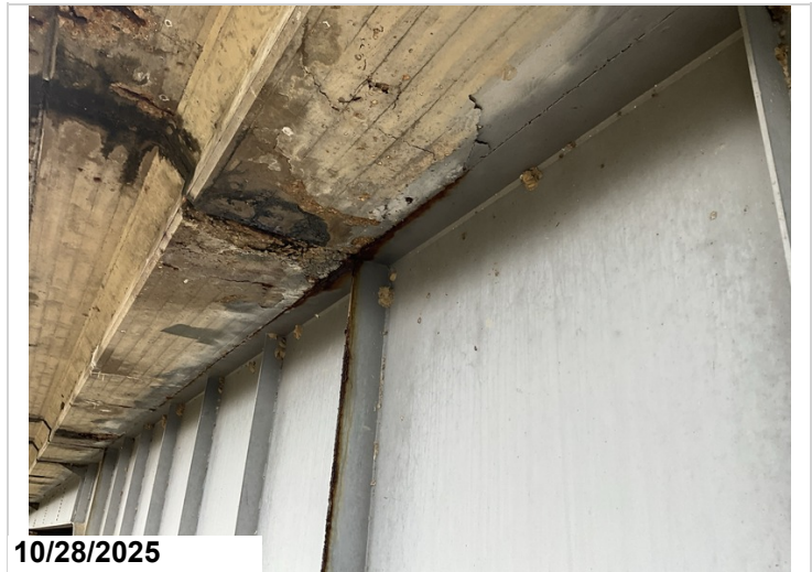
Span 9, Girder 1, Left, at third saw joint: Active corrosion with flaking rust along the Top Flange. 6LF CS3 corrosion.
