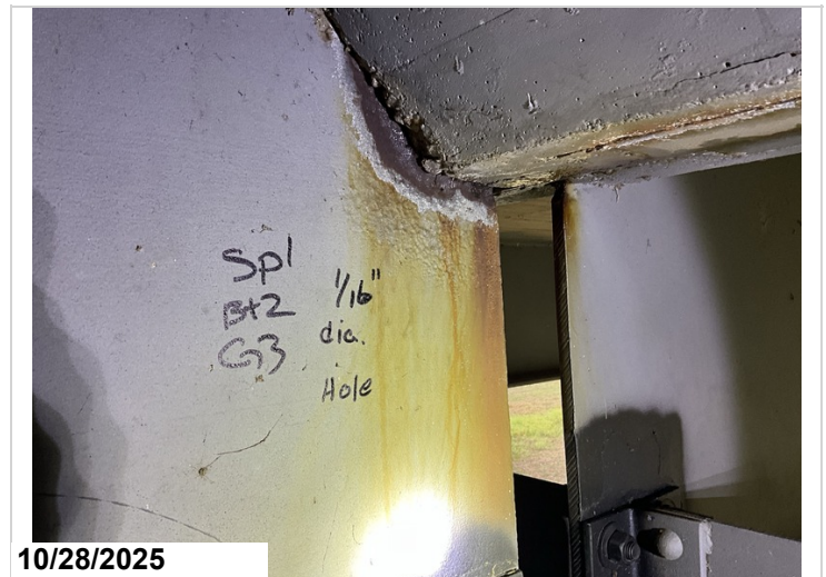
Span 1, Bent 2, Girder 3: Active corrosion with a 1/16" diameter hole in the web at the haunch area. 1LF cs4.
