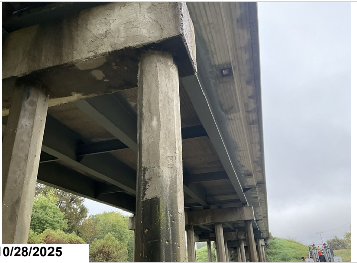
Bent 5, Pile 1: Repair. 1EA CS2 Patched area.
