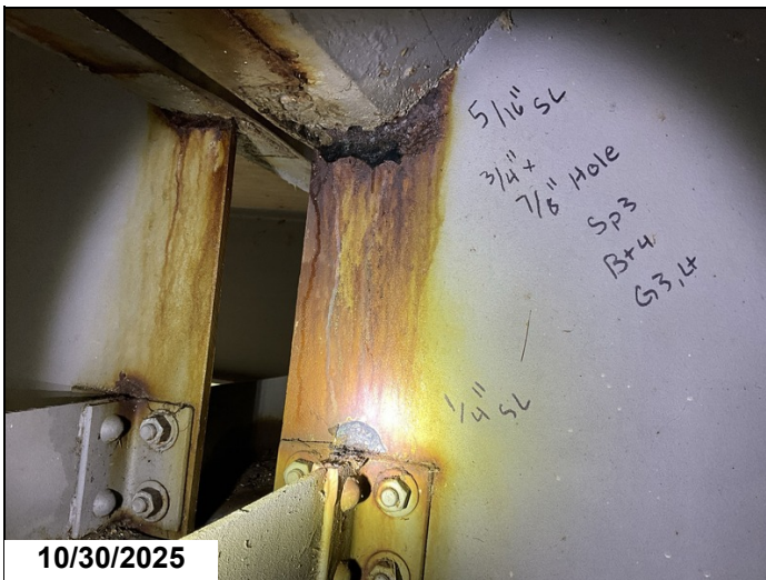
Span 3, Bent 4, Girder 3, Left: Active corrosion with section loss up to 5/16" to the web at the haunch area, a 3/4" X 7/8" hole in the web at the haunch area, and section loss up to 1/4" to the web at the diaphragm connection. 1LF CS4 corrosion.
