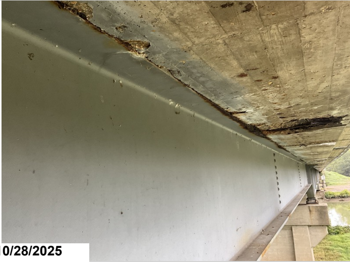
Span 6, Girder 4, Right, from joint at Bent 6 to joint at Pin and Hanger Assembly: Active corrosion with flaking rust along the Top Flange. CS3 corrosion.
