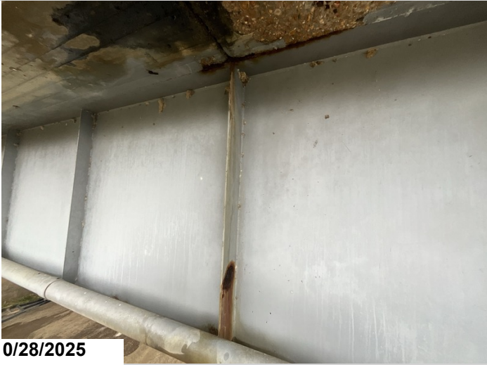
Span 9, Girder 1, Left, at second saw joint: Active corrosion with flaking rust along the Top Flange and corrosion to vertical stiffener. 3LF CS3 corrosion.
