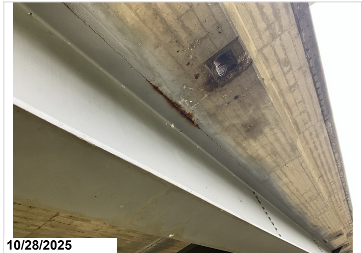
Span 2, Girder 4, Right, Top Flange: Active corrosion with flaking rust along the Top Flange. 6LF CS3 corrosion.
