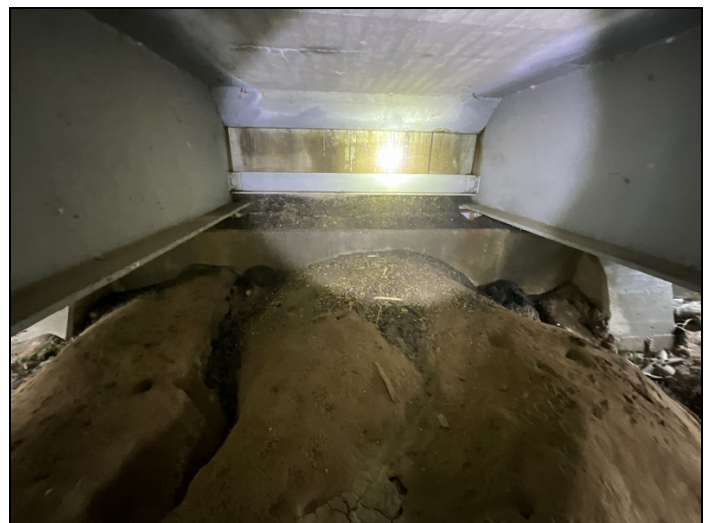
Bent 1: Cap needs cleaned.
