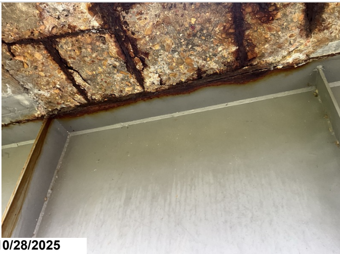
Span 7, Girder 4, Right: Active corrosion with flaking rust along the Top Flange. 21LF CS3 corrosion.
