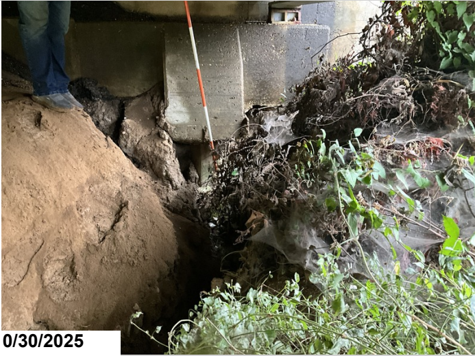
Bent 1: Erosion up to 2' below the bottom of the bridge seat under Girders 1 and 4, worst being under Girder 1 with undermining up to 2.5'. 6LF CS2 erosion, 10LF CS3 erosion.
